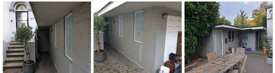
Fig. 12 Photographs of the existing garage block
