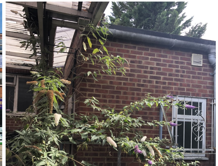
Figure 6: View of the Rear of the Site
