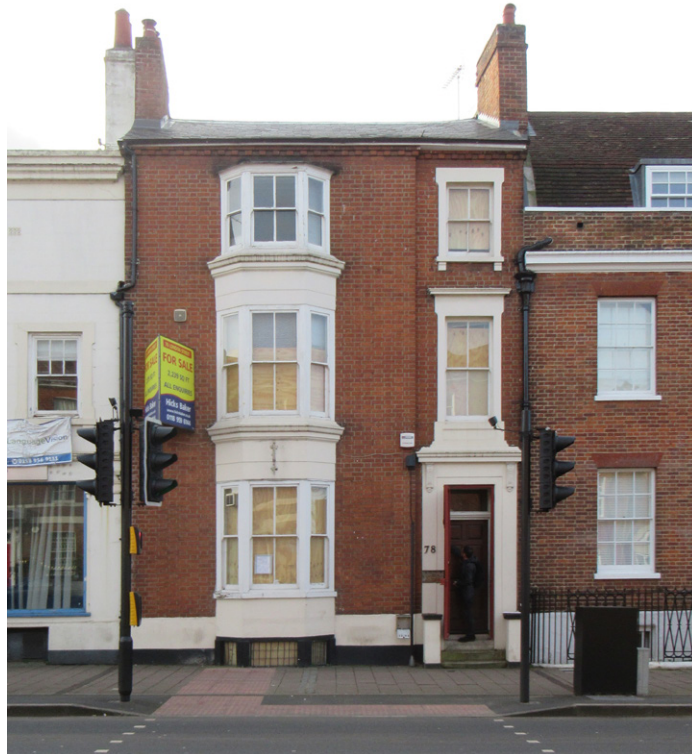
Fig 19. View of the existing London Street facade.
