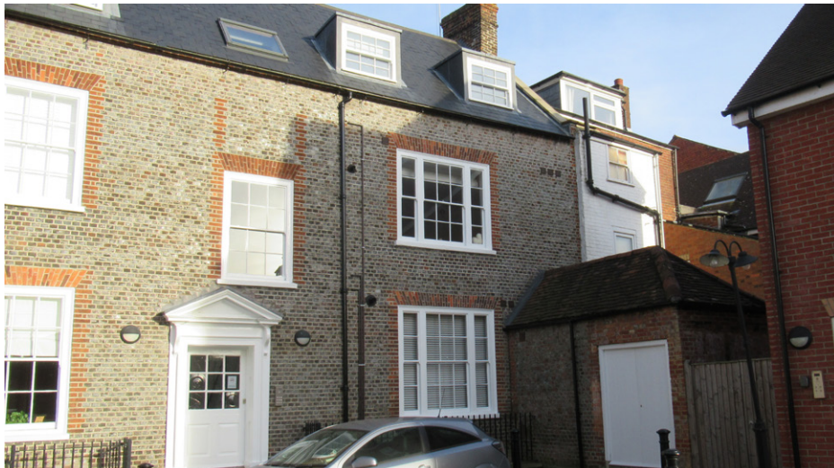
Fig.6 View from the rear parking courtyard behind no. 76 London Street
