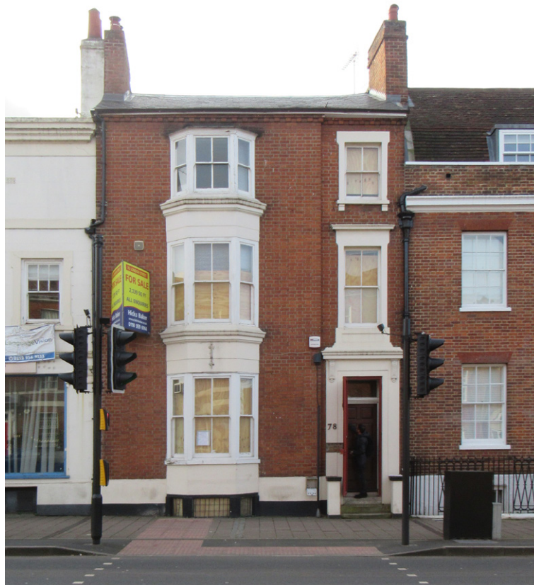
Fig 1. View of the existing London Street facade.
