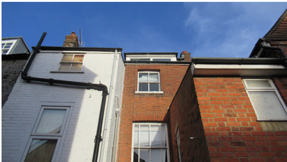
Fig.7 View of the rear facade
