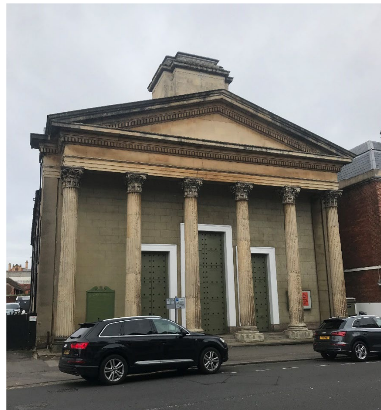
Plate 14: Grade II* Listed St Mary's Church, principal (southern) elevation viewed from Castle Street.
