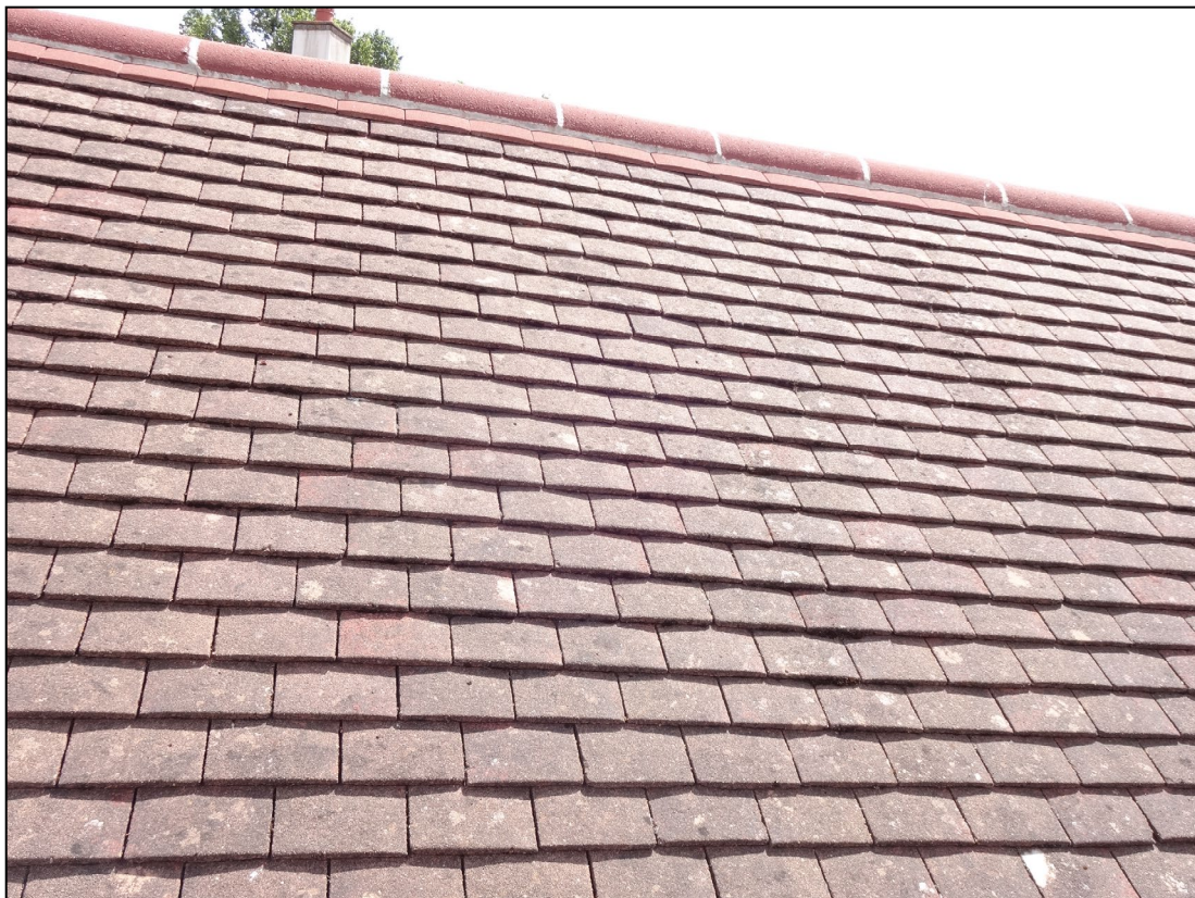
Figure 4. Example of roof structure. 3 Eric Avenue, Emmer Green. 05.06.20
