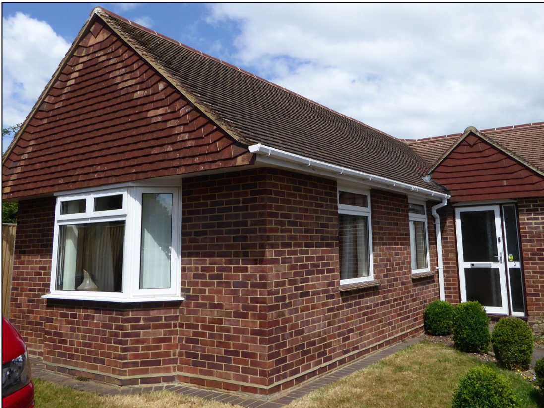
Figure 6. Well-fitting hanging tiles. 3 Eric Avenue, Emmer Green. 05.06.20
