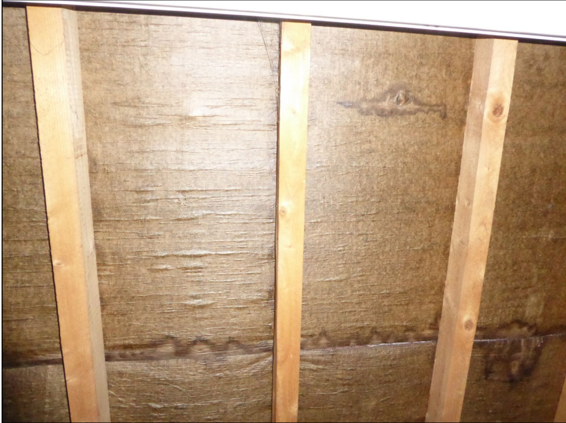
Figure 10. Tar paper lining to loft. 3 Eric Avenue, Emmer Green. 05.06.20
