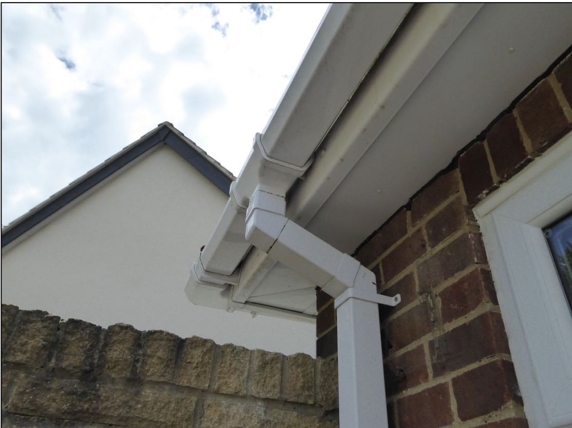
Figure 8. uPVC soffits and fascias. 3 Eric Avenue, Emmer Green. 05.06.20
