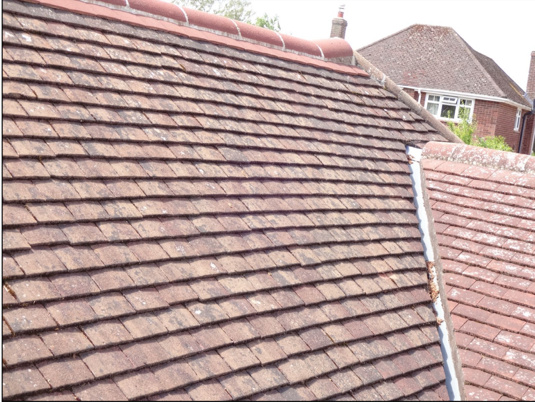
Figure 5. Example sealed ridge tiles and valleys. 3 Eric Avenue, Emmer Green. 05.06.20
