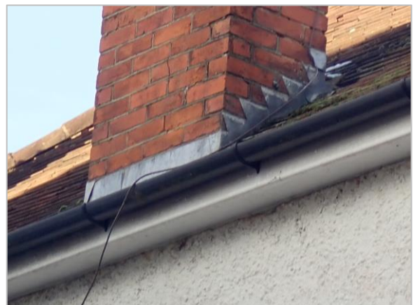
Photo 18 Chimney flashing in good condition
