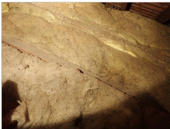
Photo 5 Loft insulation
