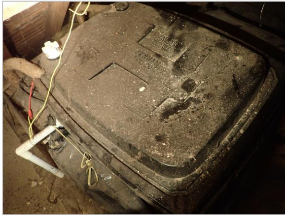
Photo 7 Top of water tank
