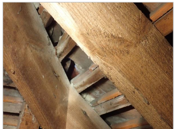
Photo 12 Timberwork below tiles
