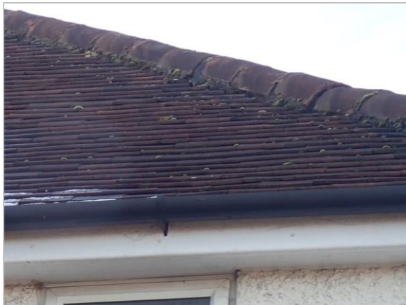
Photo 15 Roof tiles in good condition (front of house)
