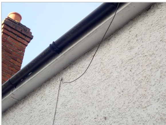
Photo 17 Soffit tight to external wall
