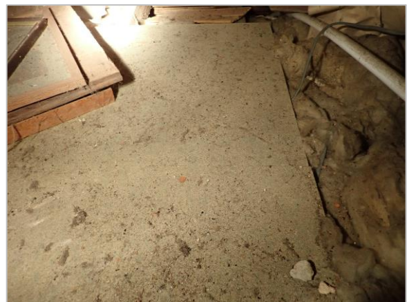
Photo 6 Loft floor boarding
