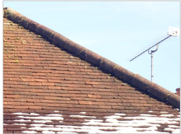
Photo 14 Roof tiles in good condition (rear of house)
