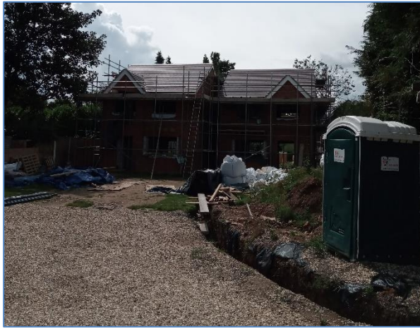
Fig 1. Three-bedroom houses (x2) under construction to the west of 4 Copse Avenue (approved under application 181306). Site photo taken by Case Officer on 09/08/2021.
