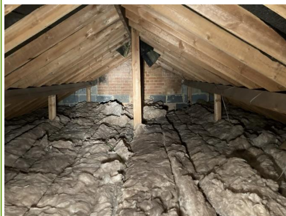
Smaller roof space
