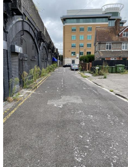
Eastern site boundary
