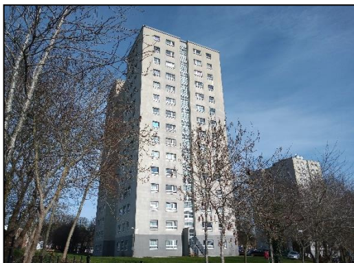
Figure 1: Photograph showing southern view of the site
