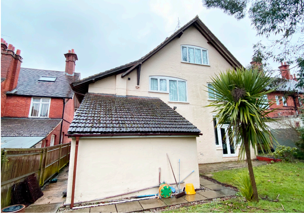
Fig.5 Existing view of the Brackenhurst Guest House rear facade
