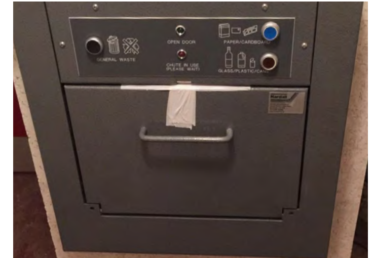
Smart Hopper with waste selection controls
