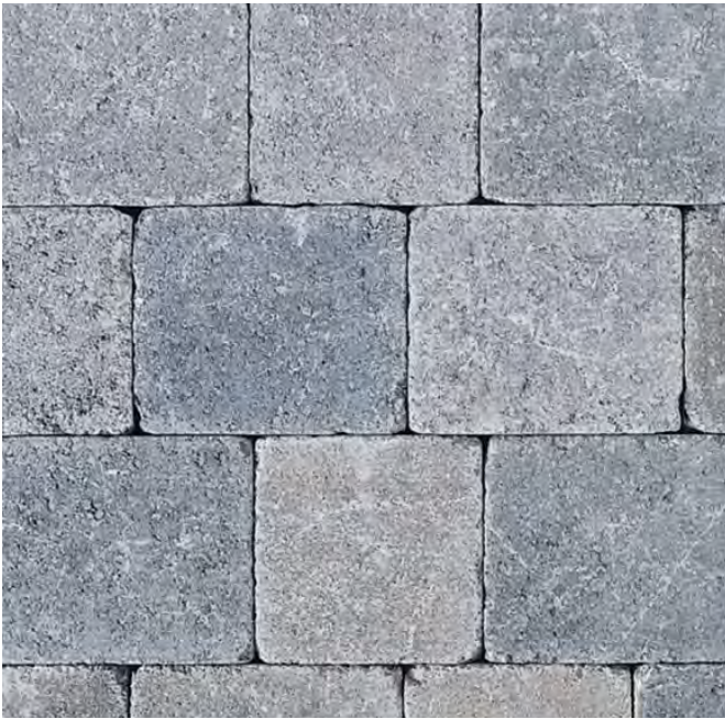
Footpaths (Phase 1) Concrete block paving
