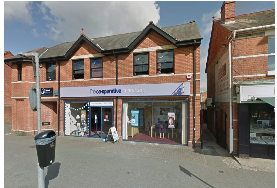
Co-operative Funeralcare, 104 School Road Large format, suspended poster signage within shopfront window. Non-illuminated.
