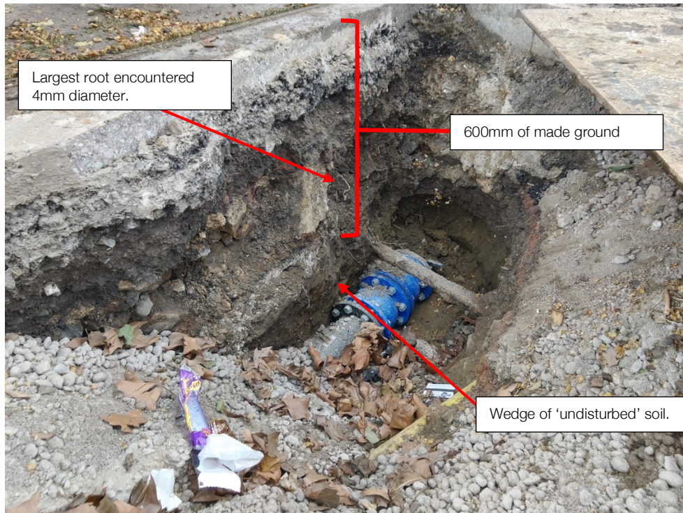
Image 2: Looking at the western face of the trench excavation adjacent the connection valve.
