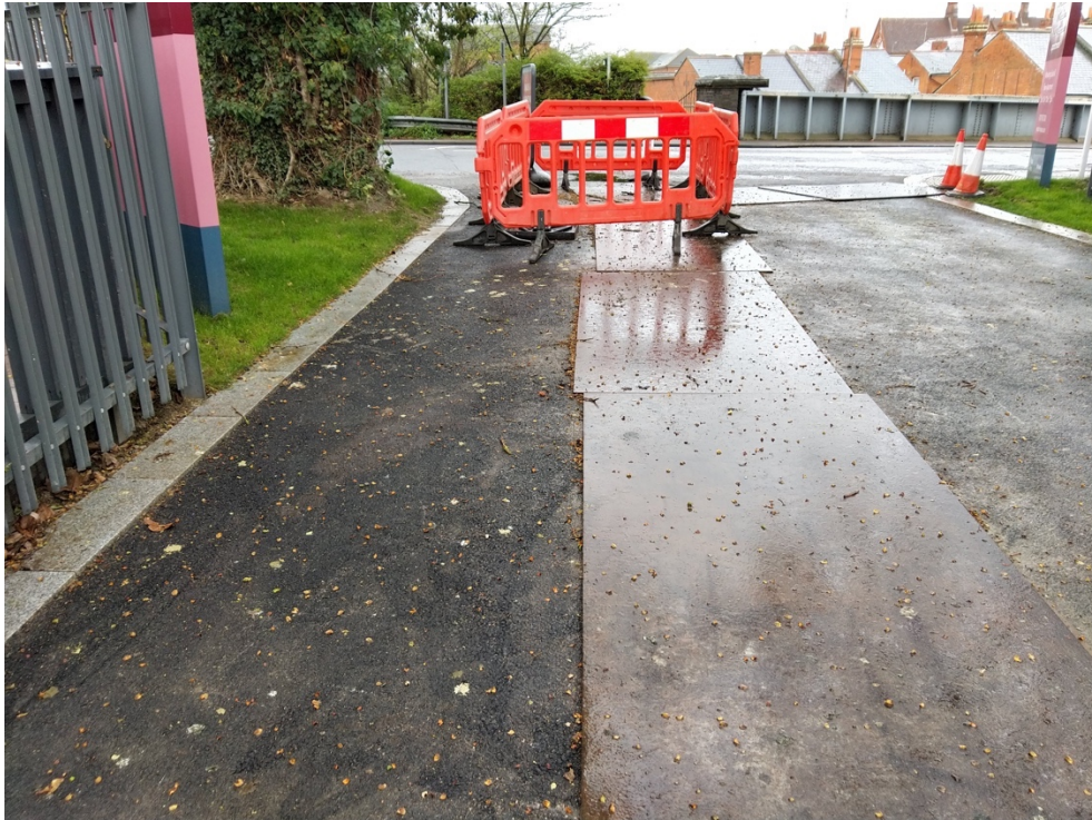
Image 1: Looking north towards Berkeley Avenue from within the site. The trench is located beneath the road plates and the subject London Plane is located to the left of frame.
