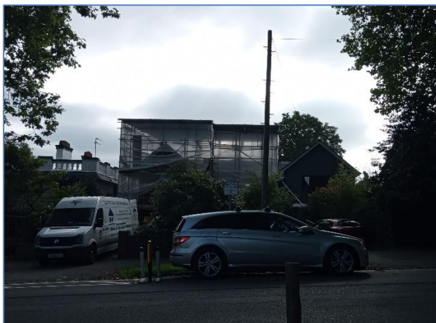
1. Front of 51 Kendrick Road. Photo taken on 14/07/2021.
