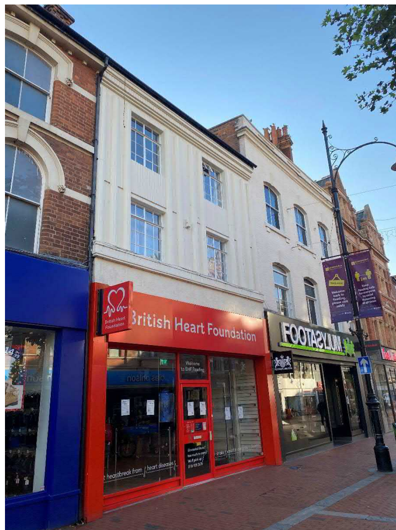
Photo 5: Broad Street façade of No 85
