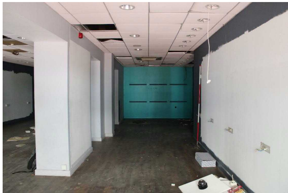
Photo 13: View south along western side of retail unit accessed from No 88, which is the ground floor of part of No 87
