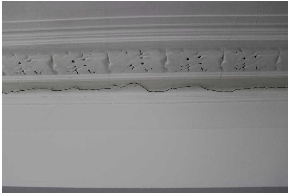
Photo 30: Surviving element of coving in western half of first floor front room fronting Broad Street
