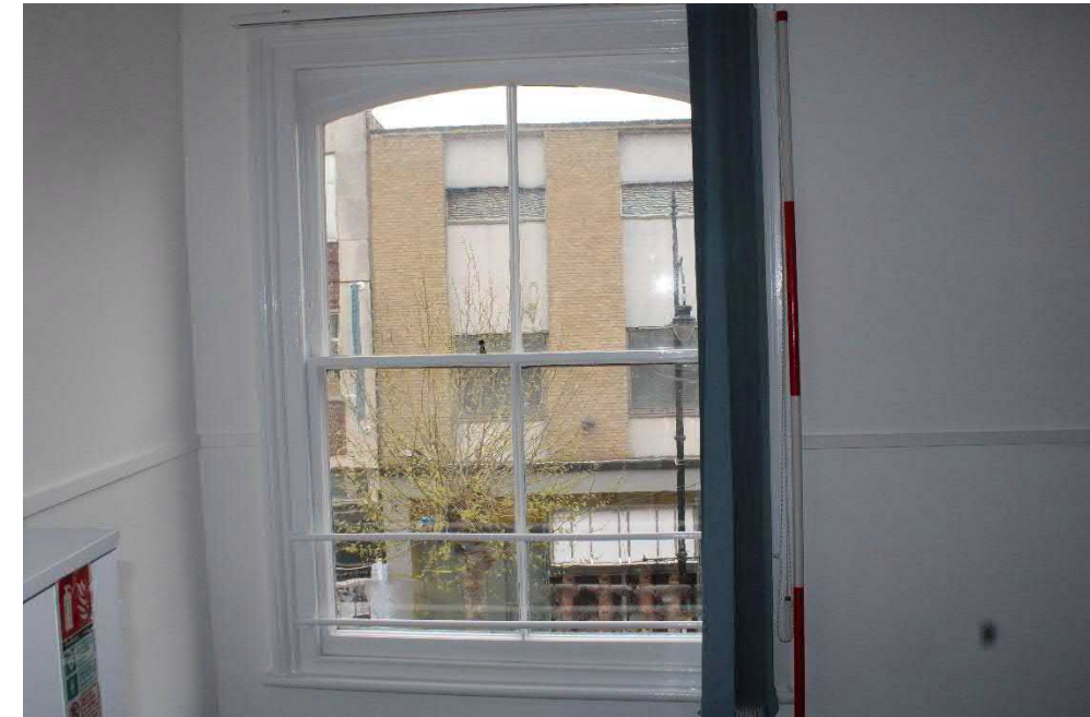
Photo 51: View north of western window of second storey room overlooking Broad Street frontage
