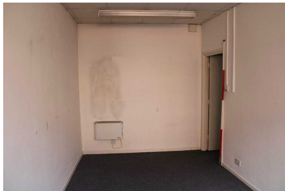
Photo 71: View south across eastern room at first floor level with doorway leading to landing area
