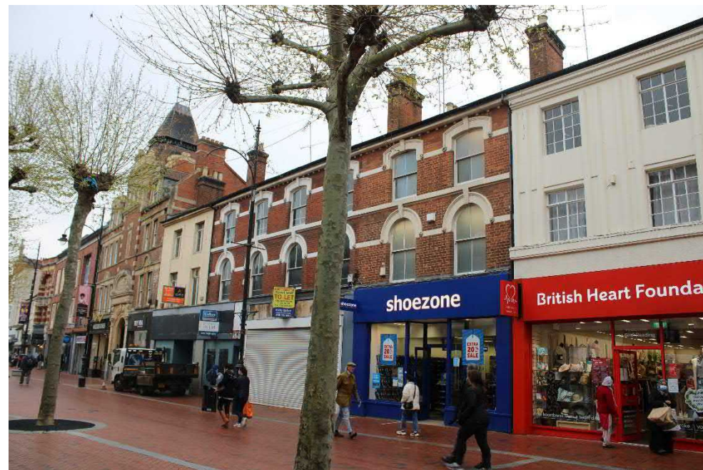
Photo 1: View southeast across the Broad Street facade of Nos 86 and 87 with red brick frontages with former elements of the original terrace (No 85 to right and No 88 to left) with later square headed windows and rendered facades
