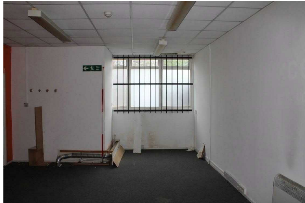
Photo 73: View south across western room of first floor level
