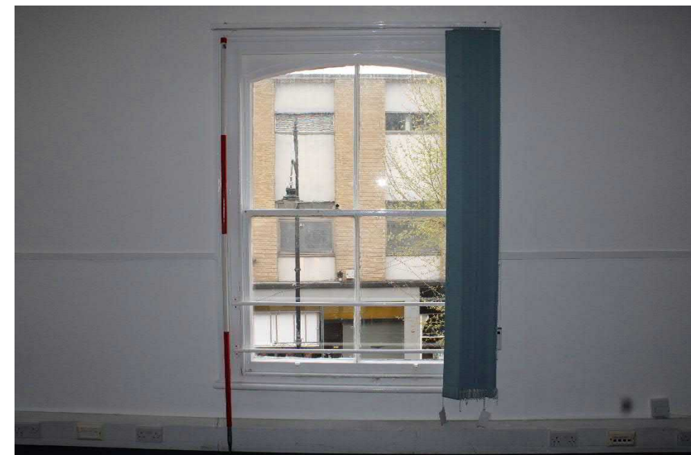
Photo 52: View north of west of centre window of second storey room overlooking Broad Street frontage
