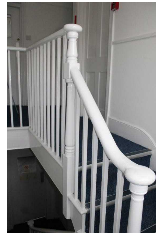
Photo 39: Detail of banisters at top of staircase leading to second floor
