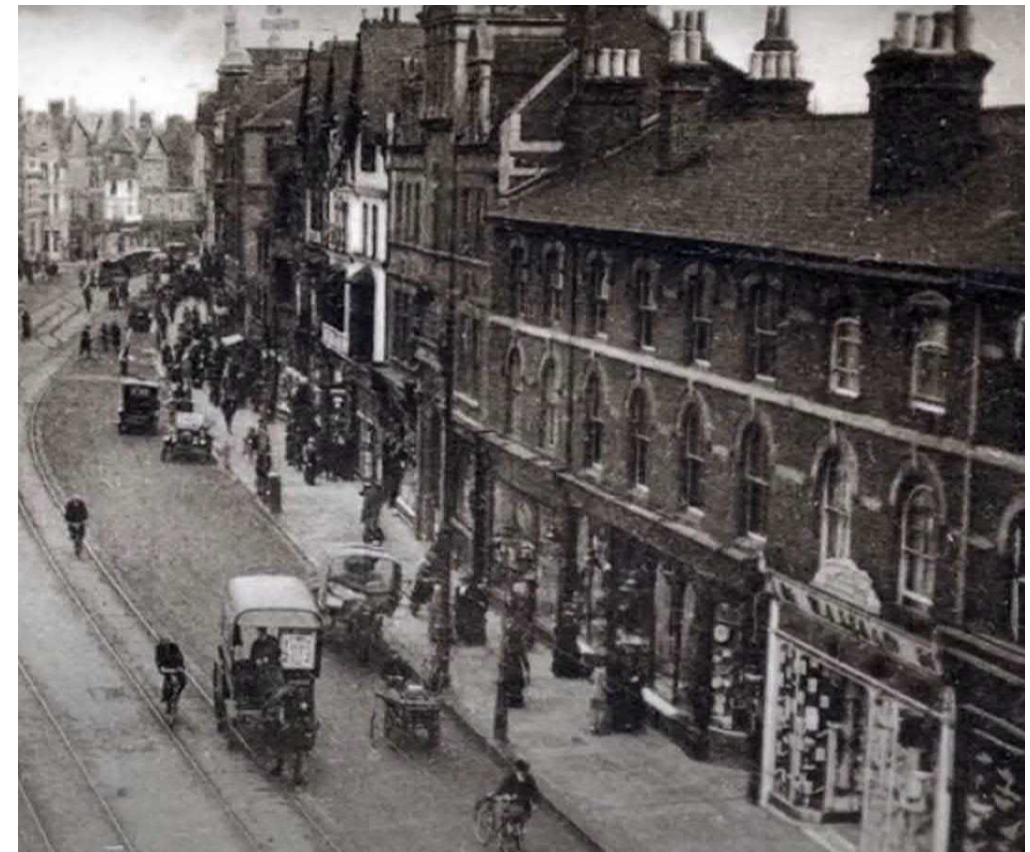
Figure 11: Historic photograph (early 20 th century) showing the application site – including Nos 88, 87, 86 and 85 (on right hand edge) as a matching terrace
