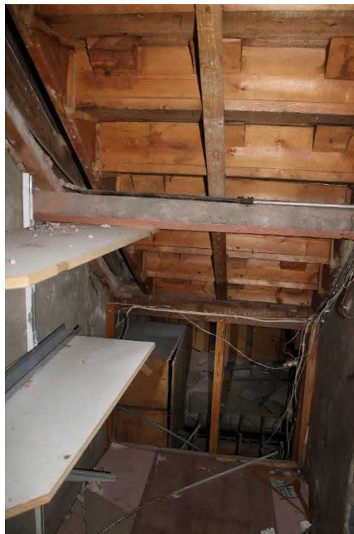
Photo 65: View west of cupboard under stairs
