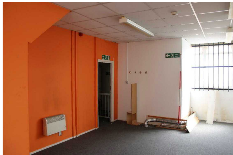
Photo 74: View southeast across western room at first floor level to landing area
