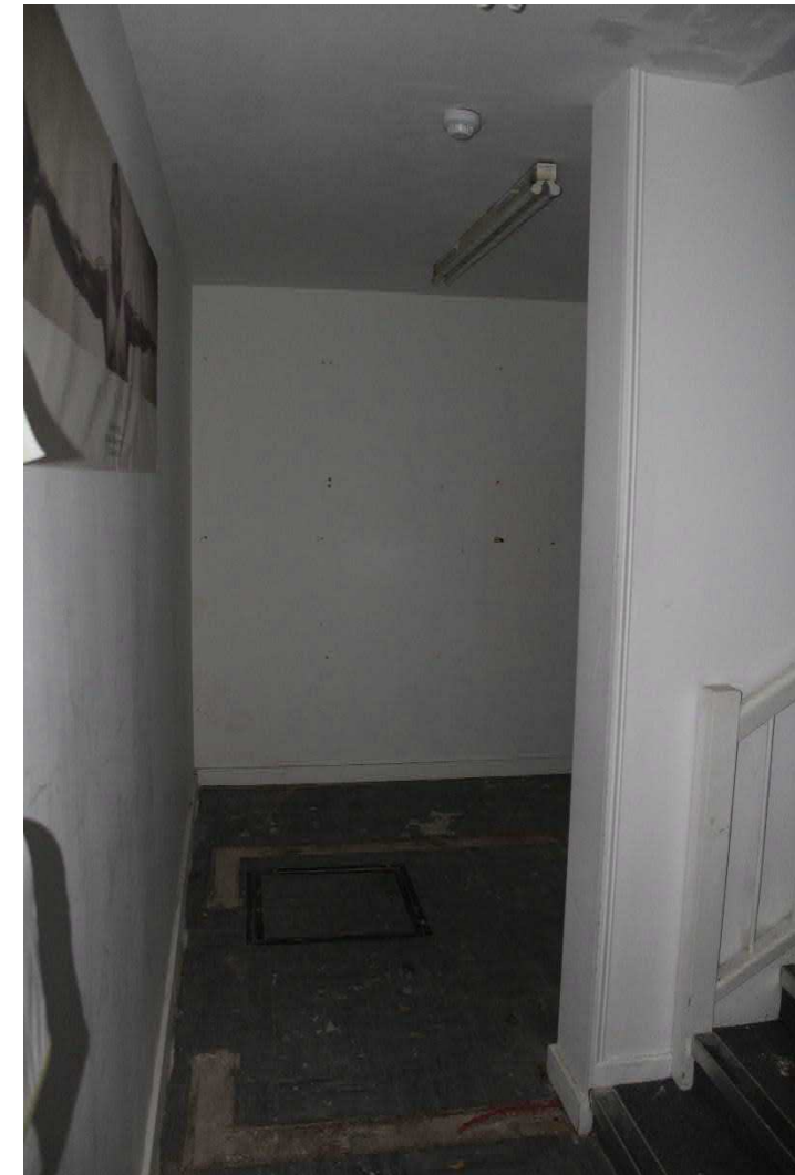
Photo 63: View east across foot of stairs showing trap door to small cellar area (not accessed)
