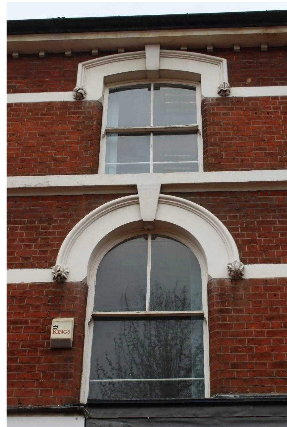
Photo 4: Detail of window arrangement on upper part of Broad Street façade, with round headed, 3-light sash window to first floor and swept head 4-light sashes to second floor. Also visible are the projecting hood moulds and vegetal label stops.
