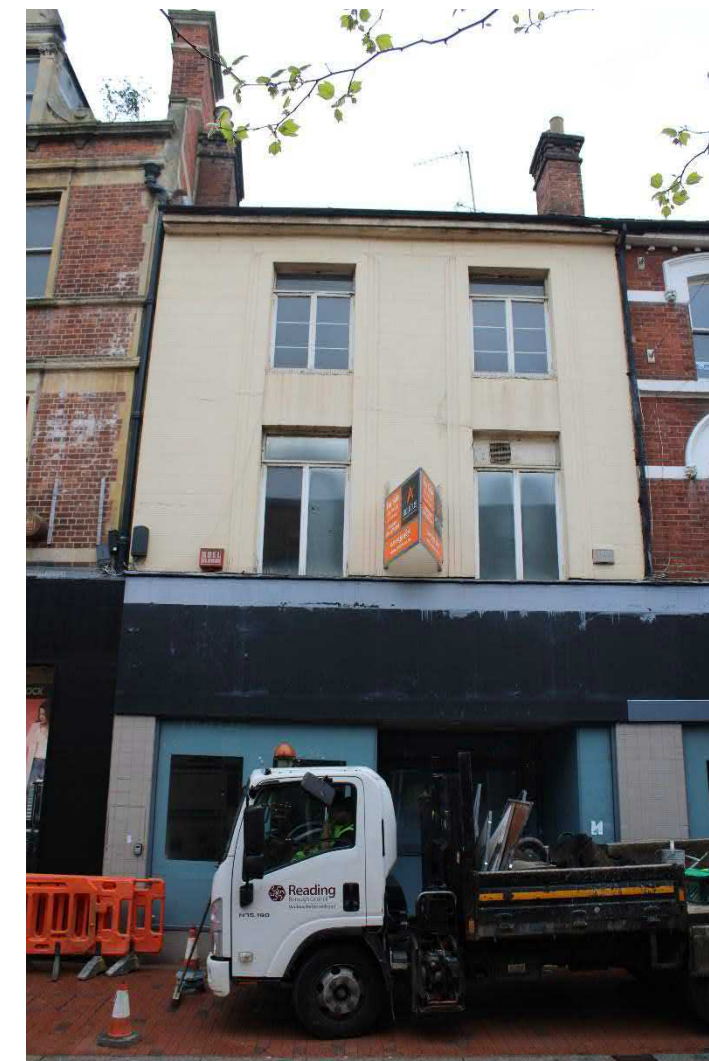
Photo 6: Broad Street façade of No 88
