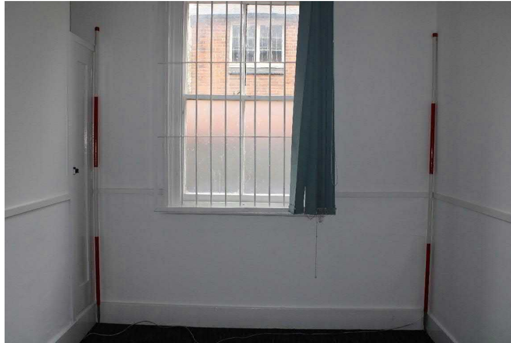
Photo 22: View south across eastern room leading off entrance vestibule with window to south elevation and three storey rear building visible through it
