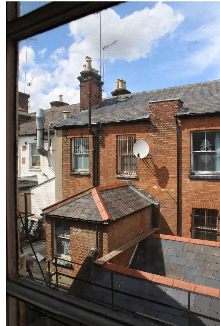
Photo 11: View northwest from second floor of three storey building to rear of No 87 showing the western half of its southern elevation, including projecting toilet block and part of the rear of No 86
