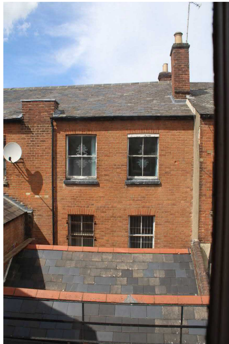
Photo 10: View north from second floor of three storey building to rear of No 87 showing the eastern half of its southern elevation
