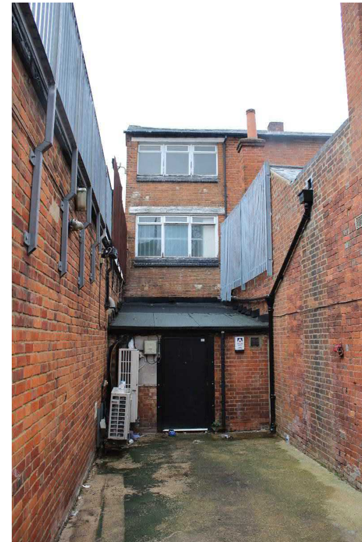
Photo 8: View north along passageway leading to rear ground floor door of No 87 located in modern extension, with later 19 th century building visible behind and with the modern store room for No 86 to left and the former school room for the chapel to the right
