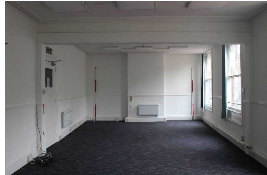
Photo 25: View west across front room of first floor of No 87 towards chimney breast, with former dividing wall location visible in foreground
