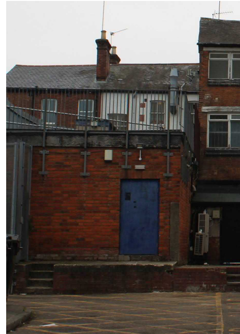
Photo 9: View of part of rear elevation of No 86 Broad Street, with single storey modern extension in front
