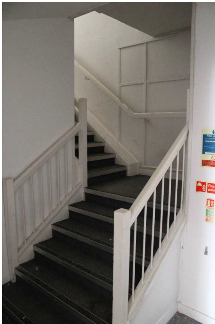
Photo 62: View of stairs on ground floor of three storey rear extension looking southeast
