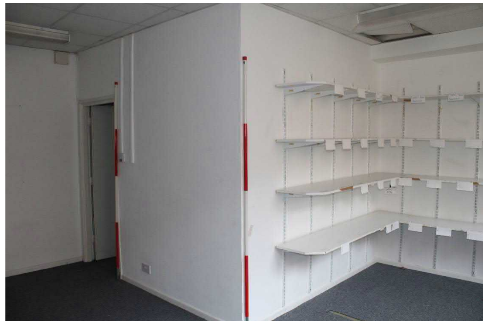
Photo 70: View southwest across eastern room at first floor level with doorway leading to landing level
