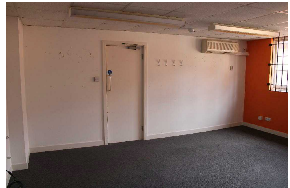
Photo 85: View west through eastern office at second floor level
