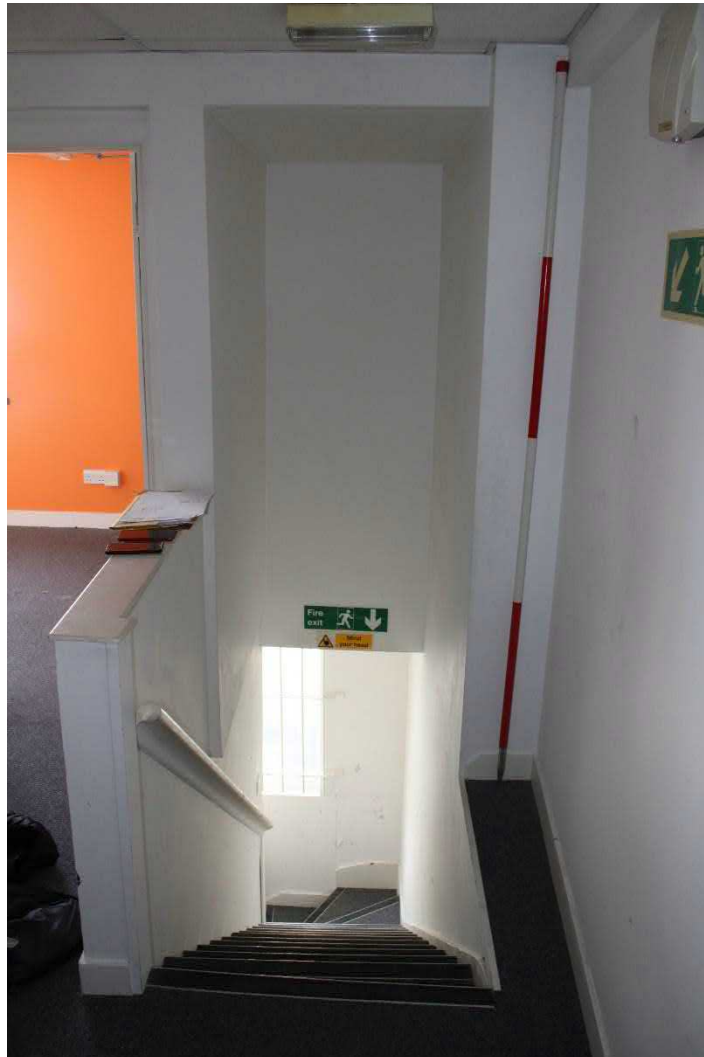
Photo 76: View north from second floor landing down the stairwell to first floor level
