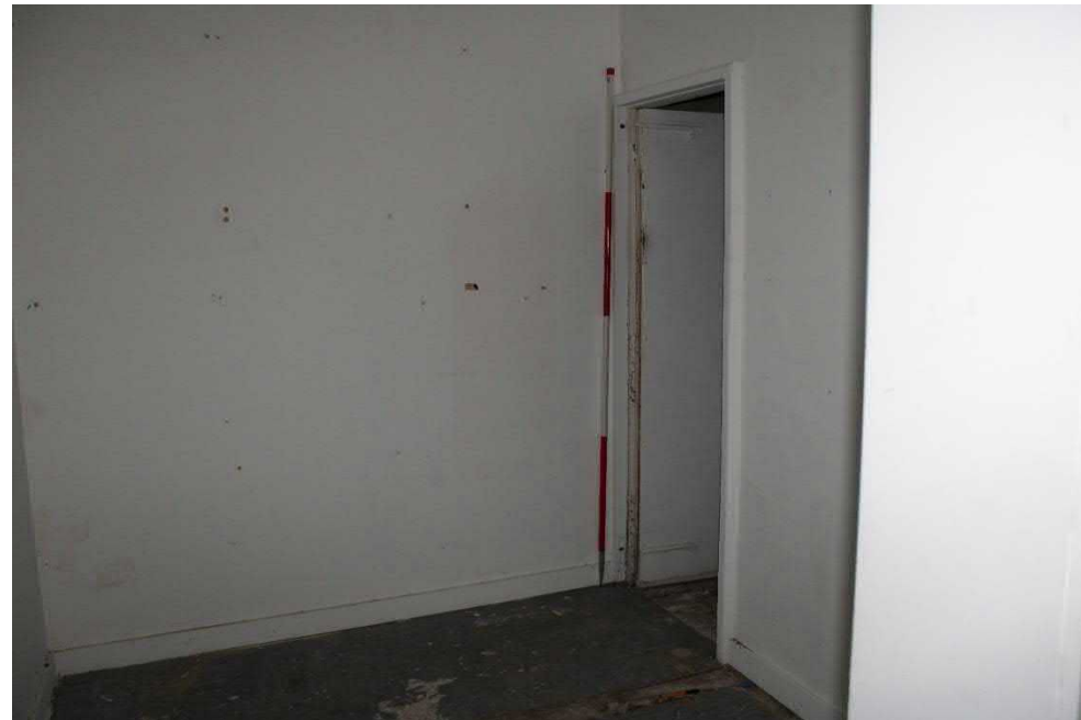
Photo 64: View southeast of entrance to cupboard below stairs
