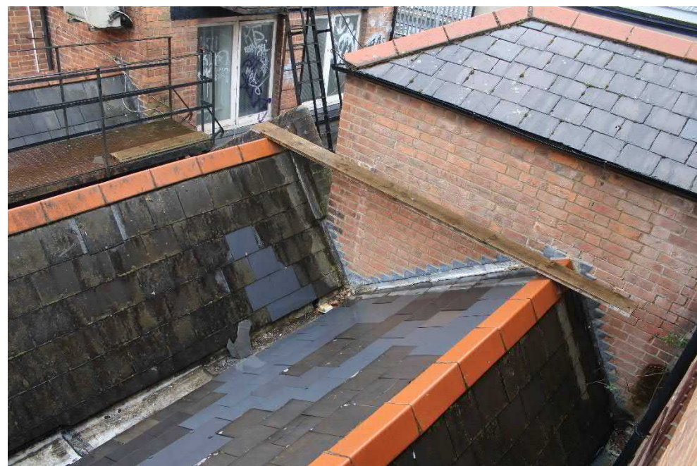
Photo 60: View south from second storey rear window of southeastern room of No 87 Broad Street showing part of saw tooth roof and projecting toilet extension (not shown on a plan)
