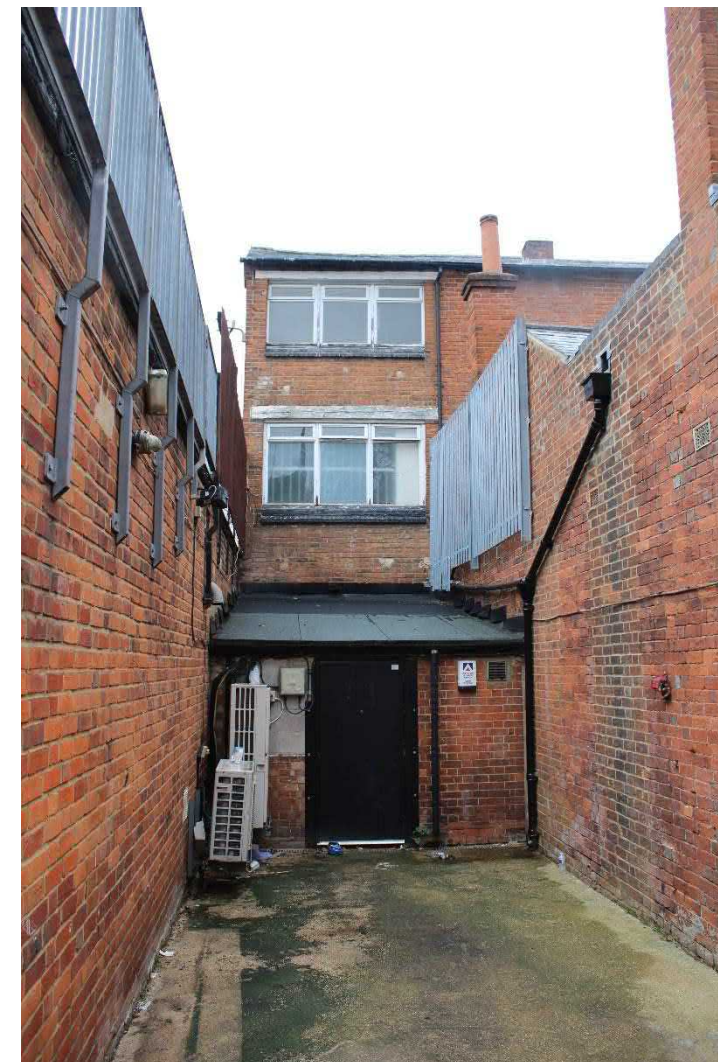
Photo 61: View north of rear part of three storey building to rear (not shown on a plan)
