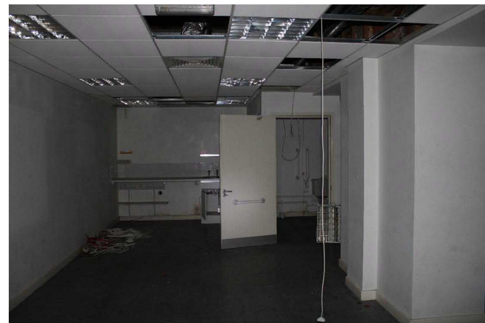
Photo 15: View north along rear room behind eastern part of shop floor with saw tooth roof line above visible through missing ceiling tiles
