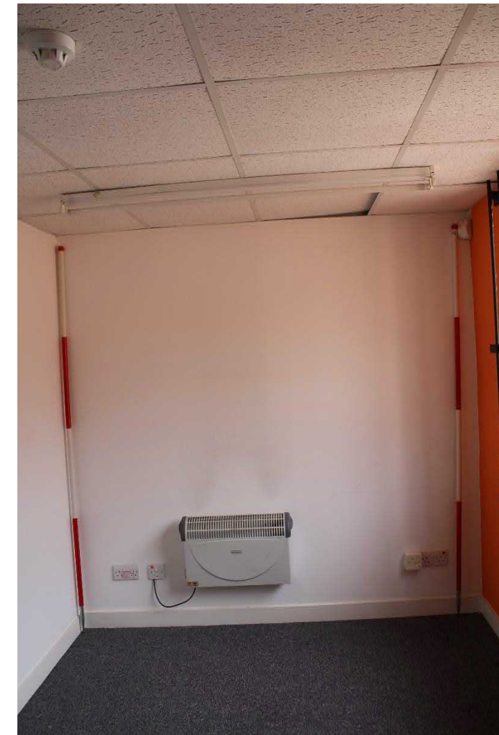
Photo 77: View west of northwestern room at second floor level
