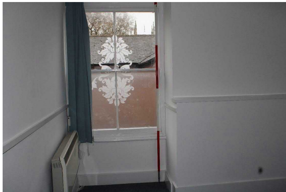
Photo 40: View south of window and end wall in room adjacent to top of stairs on second floor landing
