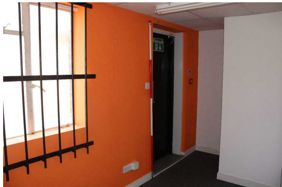
Photo 79: View northeast across northwestern room at second floor level to fire-escape doorway
