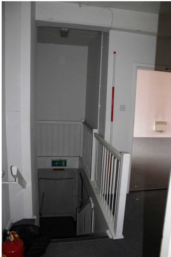
Photo 67: View west across top of stairs at first floor level across landing
