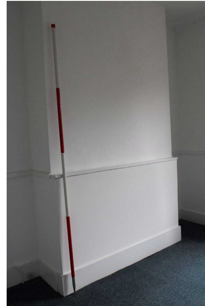
Photo 46: View southeast of chimney breast of southeastern room of No 47 Broad Street
