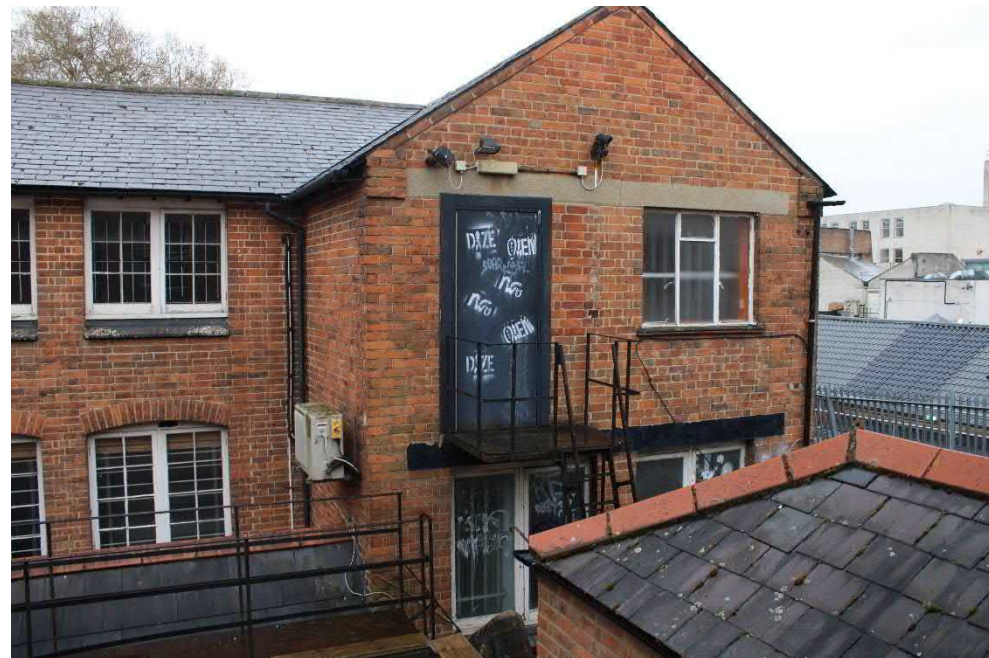
Photo 59: View south from second storey rear window of room west of stairs of No 87 Broad Street (not shown on a plan)
