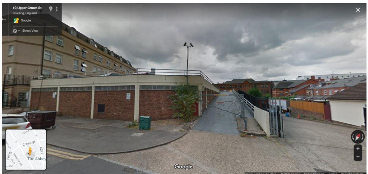
View of application site showing single storey building on western side of site with car park above (Source: Google Street View)
