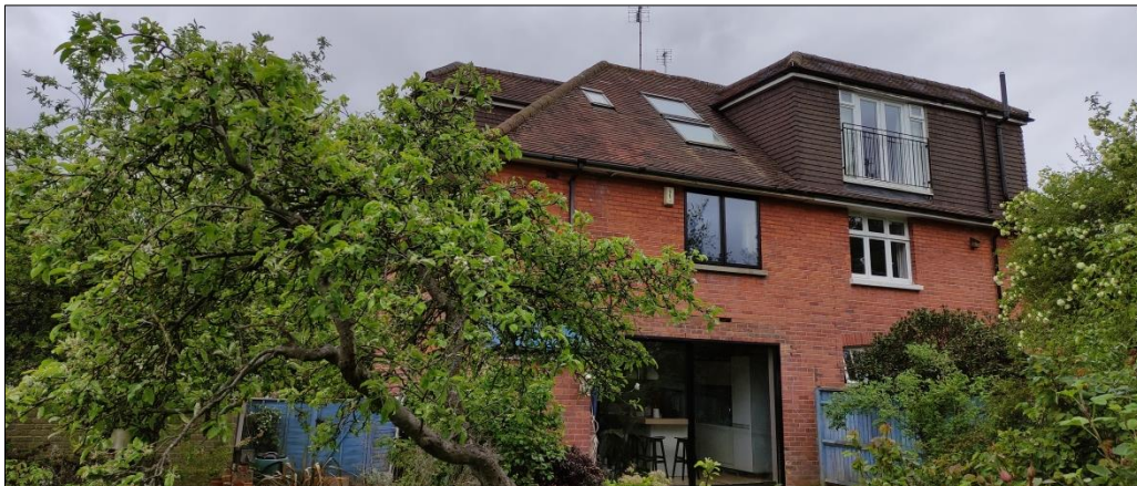
Figure 3 – Rear (northern) elevation of 87 Balmore Drive
