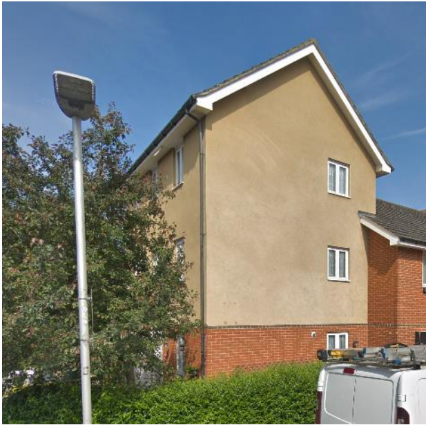
Image 7 - 16 Park View, front / flank elevation
