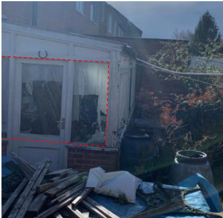
Image 5 - Rear lean-to extension at 224 Elgar Road South
