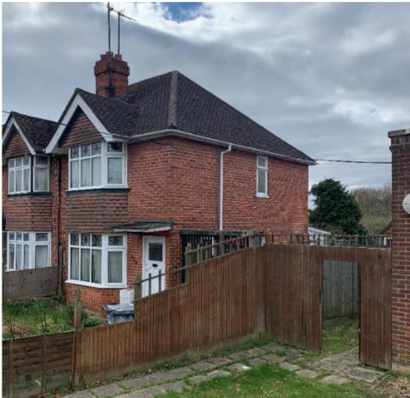
Image 4 - 224 Elgar Road South, front / side elevation
