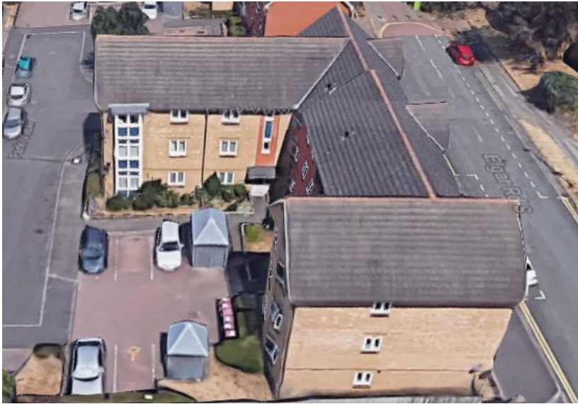
Image 3 - Aerial view of 1-12 Park View, south elevation
