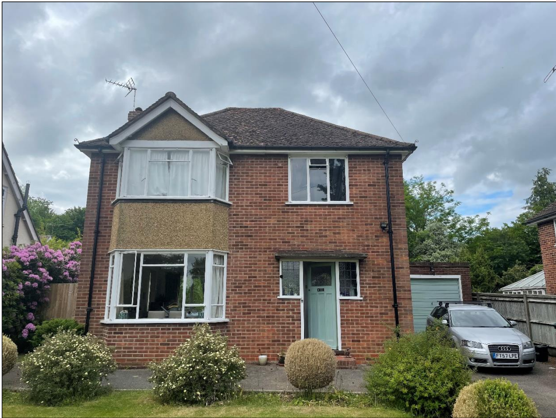
Plate 1. Front (southern) aspect of the building
