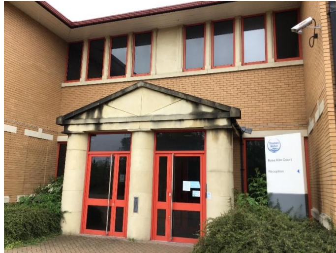
PLATE 3 SHOWING STONE ENTRANCEWAYS
