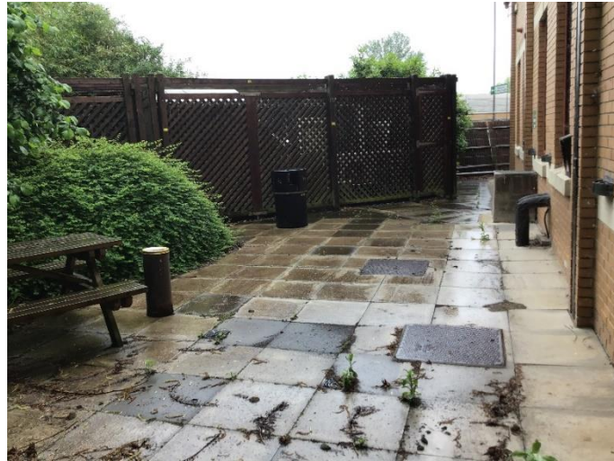
PLATE 14 SHOWING HARDSTANDING PAVING
