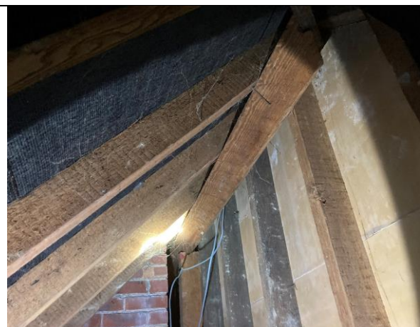
Photo 10 Old cobwebs at roof timbers
