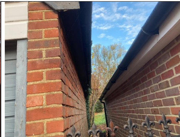
Photo 18 Sealed soffit at garage
