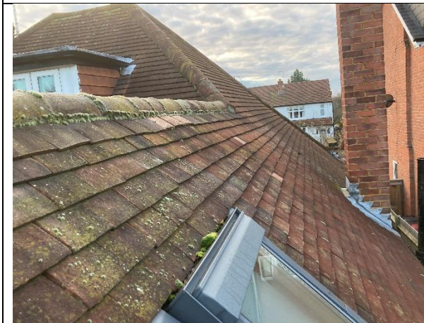
Photo 3 West hip and pitch well-sealed
