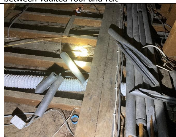
Photo 14 No evidence of bats at loft floor
