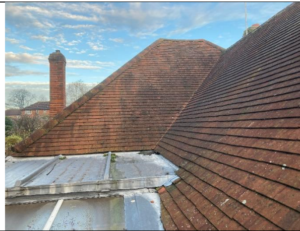
Photo 2 West pitch and south hip well-sealed
