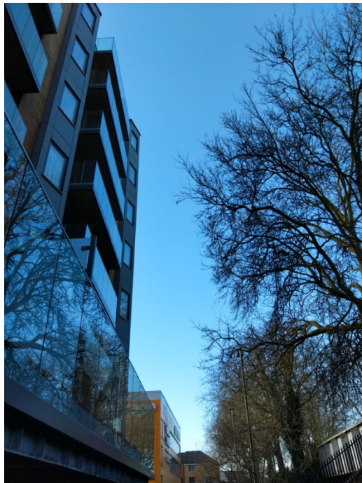
Photo 4: showing the clearance between the northern elevation the finished building and T1 now that the scaffold has been removed.
