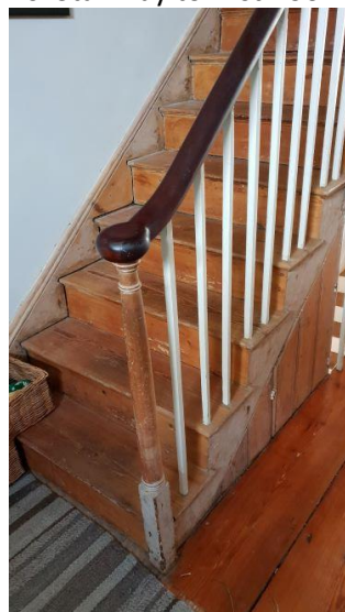
16 Stairway to first floor
