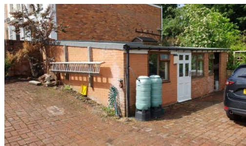
2 Brick shed at bottom of rear garden
