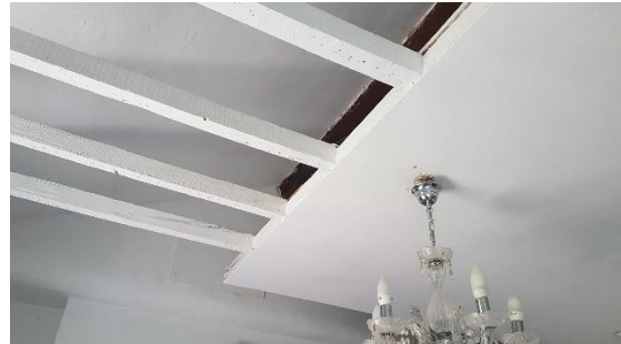
18 Repaired ceiling on original rafters rear bedroom
