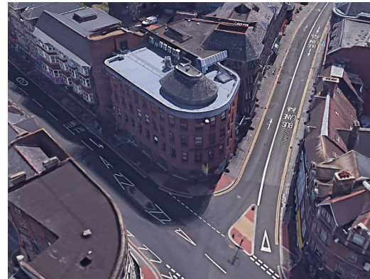
Fig 2: Aerial view towards site
