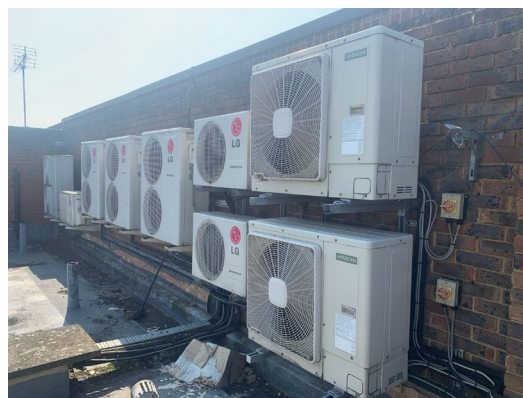
Fig 8: Existing condensers on the roof of the subject building, all to be removed except one (see Figure 9)
