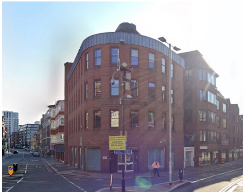
Fig 1: Site from Kings Road
