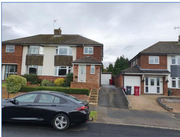
1. Front of 49 Elmstone Drive. Photo provided by the agent on 07/12/2020.
