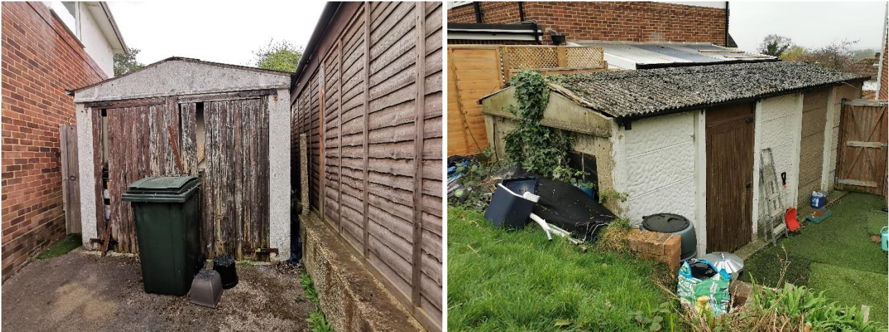
Figure 8. View of the detached garage on site
