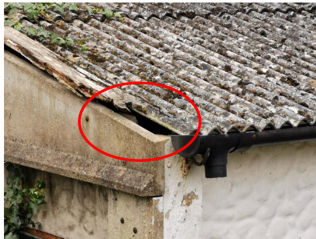
Figure 9. View of the potential access point into the garage
