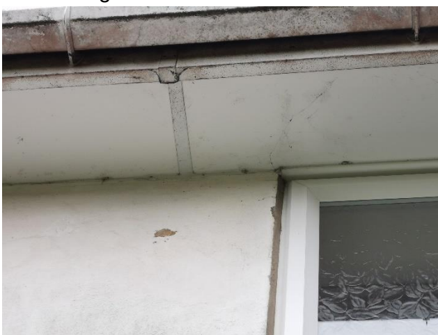
Figure 6. Example of tightly fitted soffit
