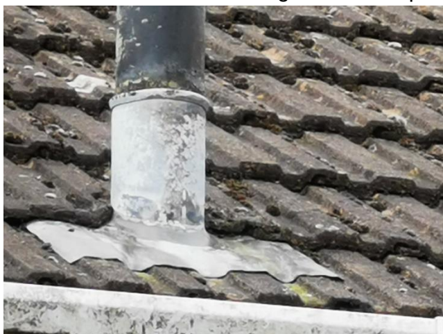
Figure 7. View of the lead flashing around the base of the flue and chimney
