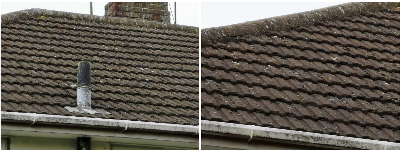
Figure 4. Example of roof tiles in a good condition
