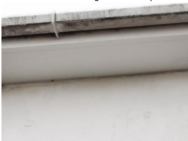
Figure 6. Example of tightly fitted soffit
