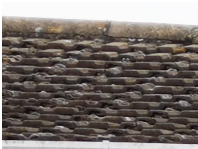
Figure 5. Example of roof tiles in a good condition
