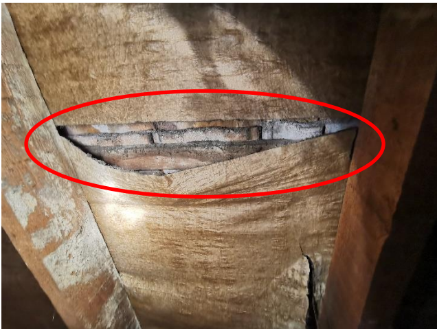
Figure 12. Example of tears/cuts in the roofing felt
