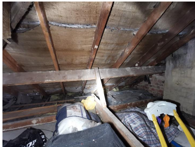
Figure 11. Internal view of the loft void
