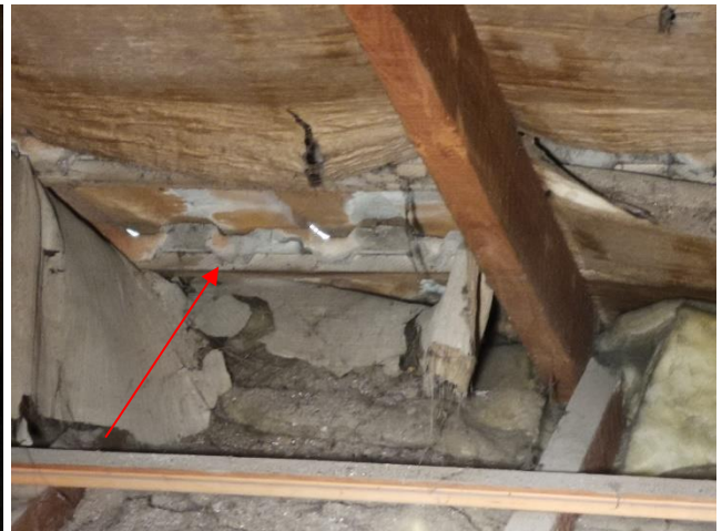
Figure 12. Example of tears/cuts in the roofing felt
