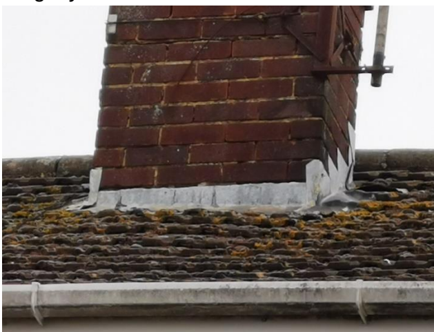
Figure 7. View of the lead flashing around the base of the flue and chimney
