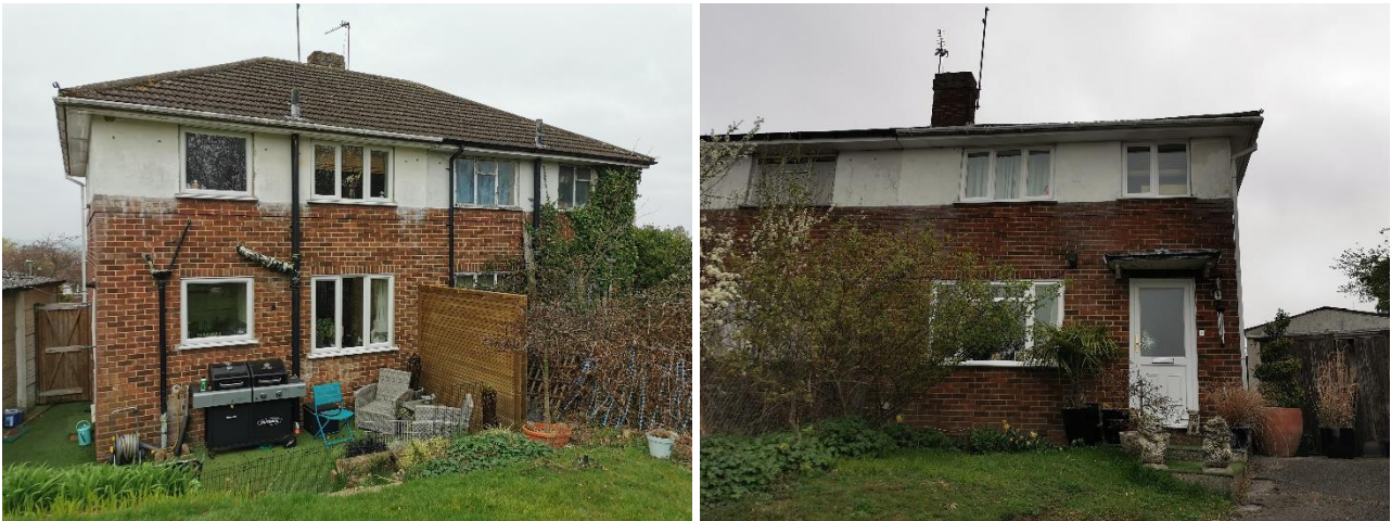
Figure 3. View of the rear/eastern (left) and front/western (right) elevations of the dwelling
