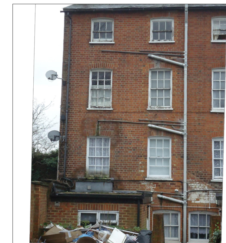
Photo of 33 Rear Elevation
