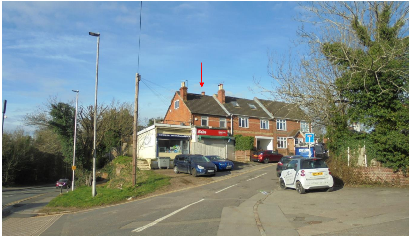
Photo 1 – Front Elevation from Bath Road
