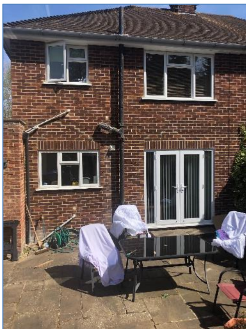
1. Rear of 10 Larkwood Close. Photo provided by the agent on 29/06/2021.
