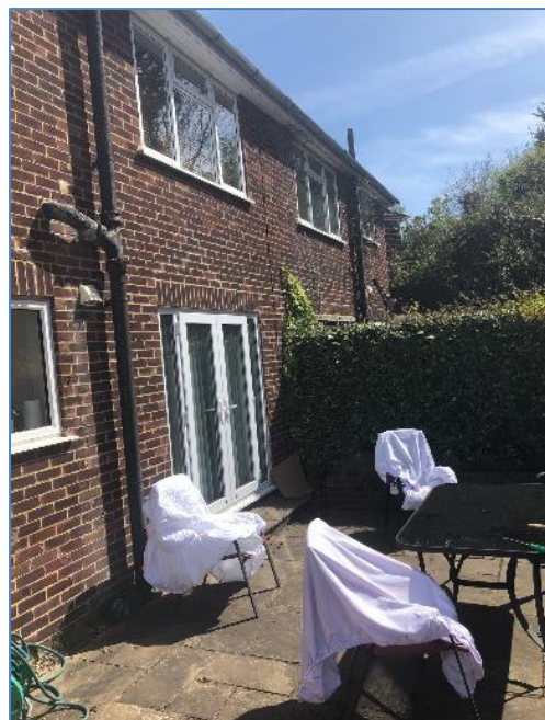
2. Rear of 10 Larkwood Close. Photo provided by the agent on 29/06/2021.
