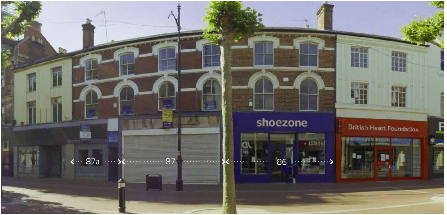
Front of the existing building from Broad Street showing the vacant retail units
