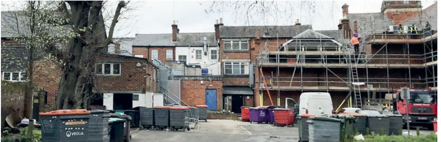
Rear of the existing building and unsightly service area, which detracts from the setting of the Reading Minster of St Mary
