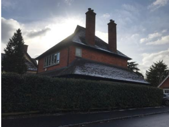
Photograph 3: North east elevation of the building
