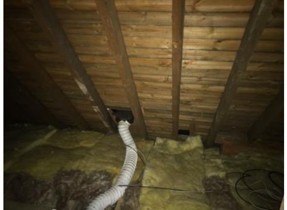
Photograph 4: Interior of loft space within the building
