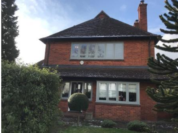
Photograph 1: East elevation of the building
