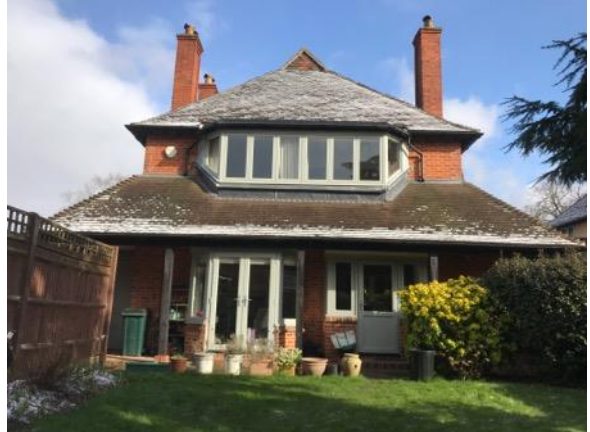
Photograph 2: West elevation of the building
