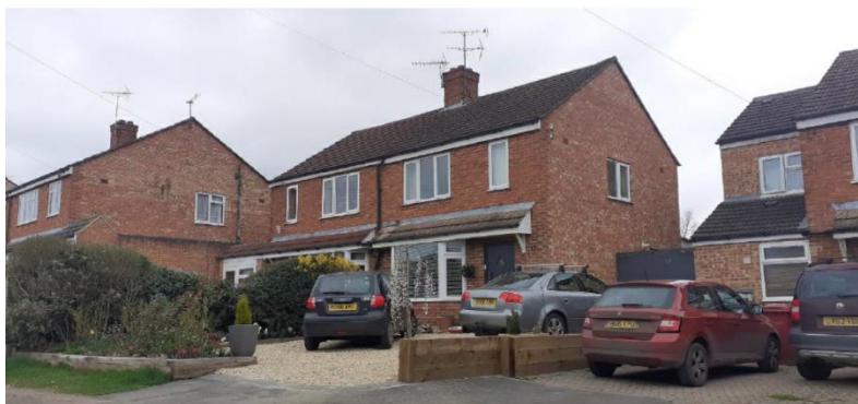
No. 33 showing gravel driveway
