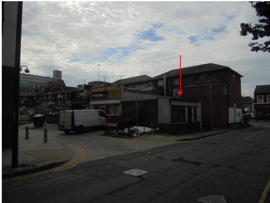
Photo 3 View on approach from Chatham Street
