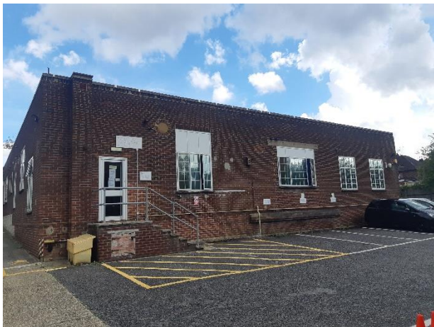
Photograph 3. The western face of the building and tarmac hard-standing car park
