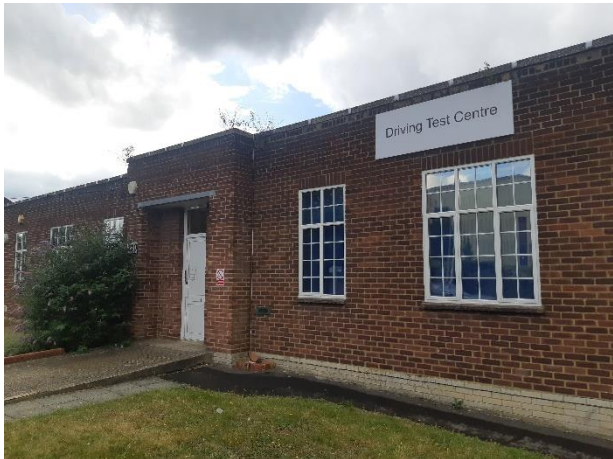
Photograph 1. The building (former driving test centre) at Elgar Road, Reading, viewed from the north-east.
