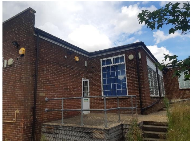
Photograph 2. The building viewed from the south-west.
