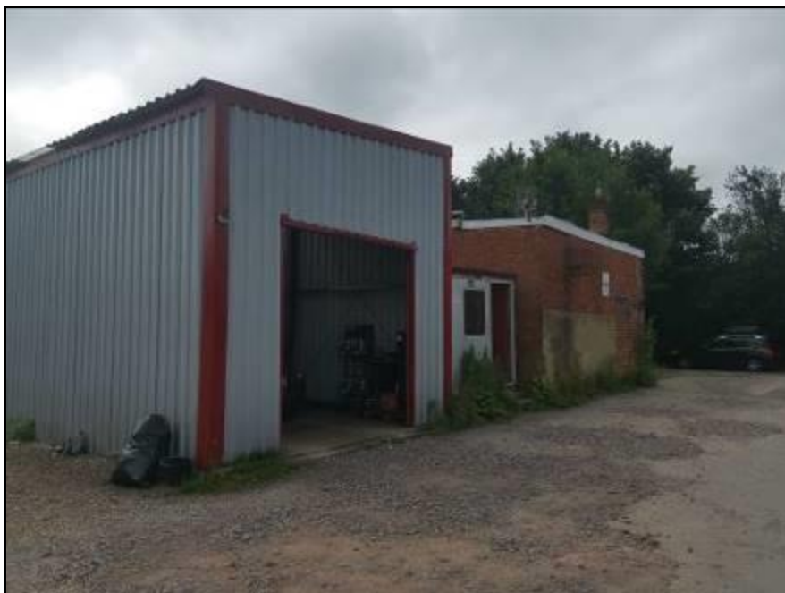
Photograph 2 Showing the motor repairs garage on the eastern section
