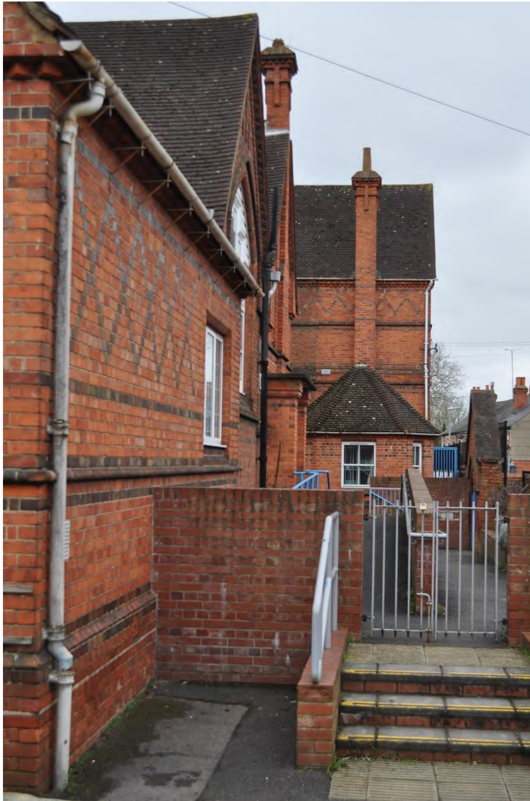
4.4.4 West Elevation 1 Brickwork and 4.5.7 Downpipes
