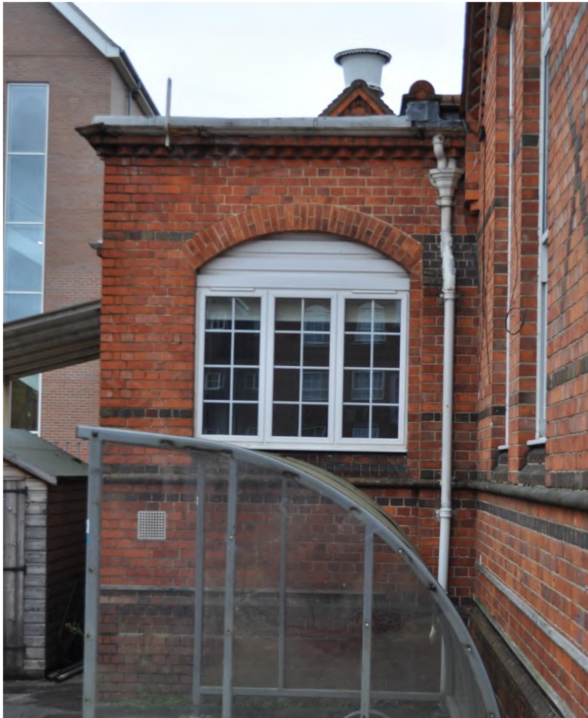
4.4.4 West Elevation 1 Brickwork, 4.5.4 Gutter, 4.5.6 Downpipes and 4.5.10 CI air bricks
