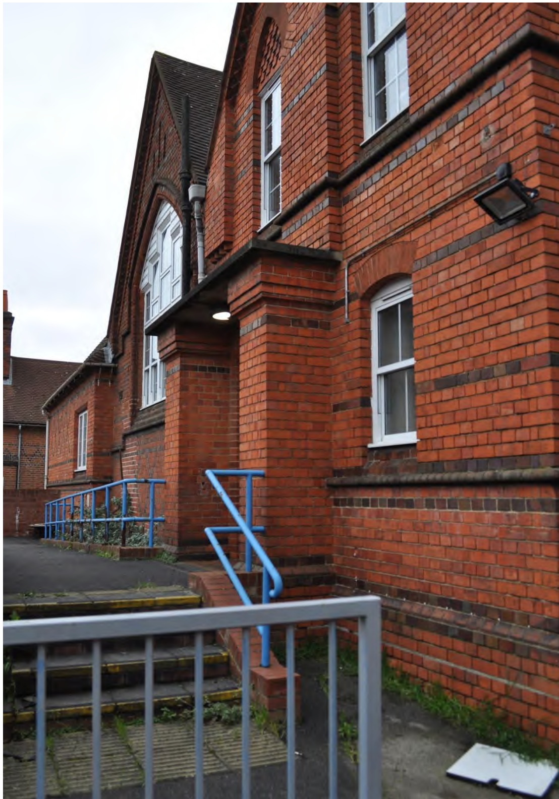
4.4.7 West Elevation 1 Brickwork
