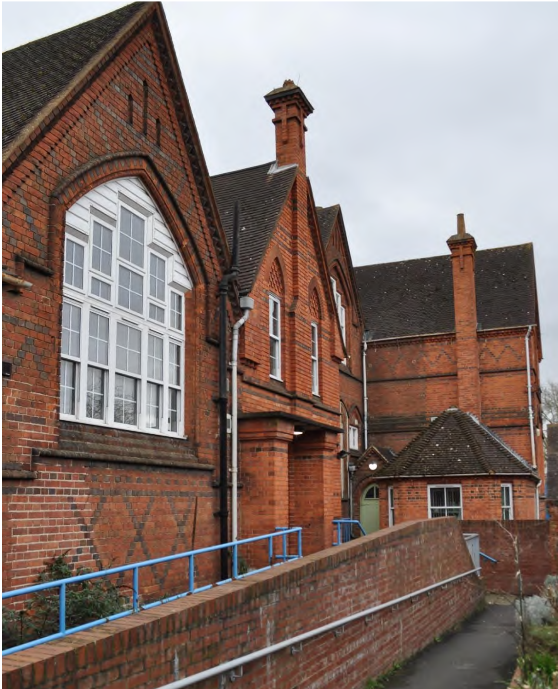
4.4.5 West Elevation 1 Brickwork and 4.5.8 -.9 Downpipes
