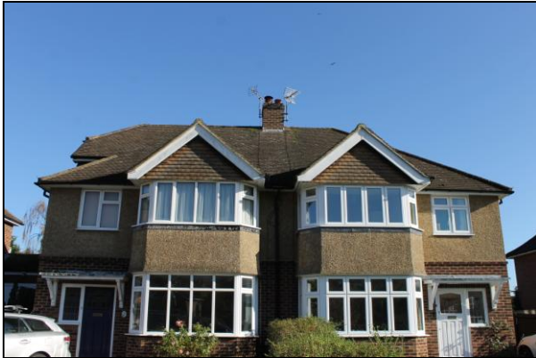
Plate 1: View of front, western elevation showing area of hanging tiles in gable
