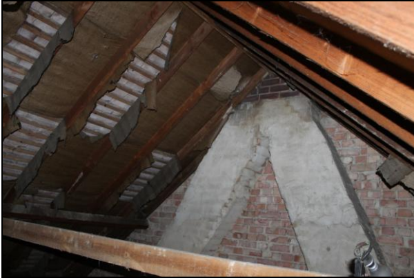
Plate 5: View of the house roof with split chimney stack
