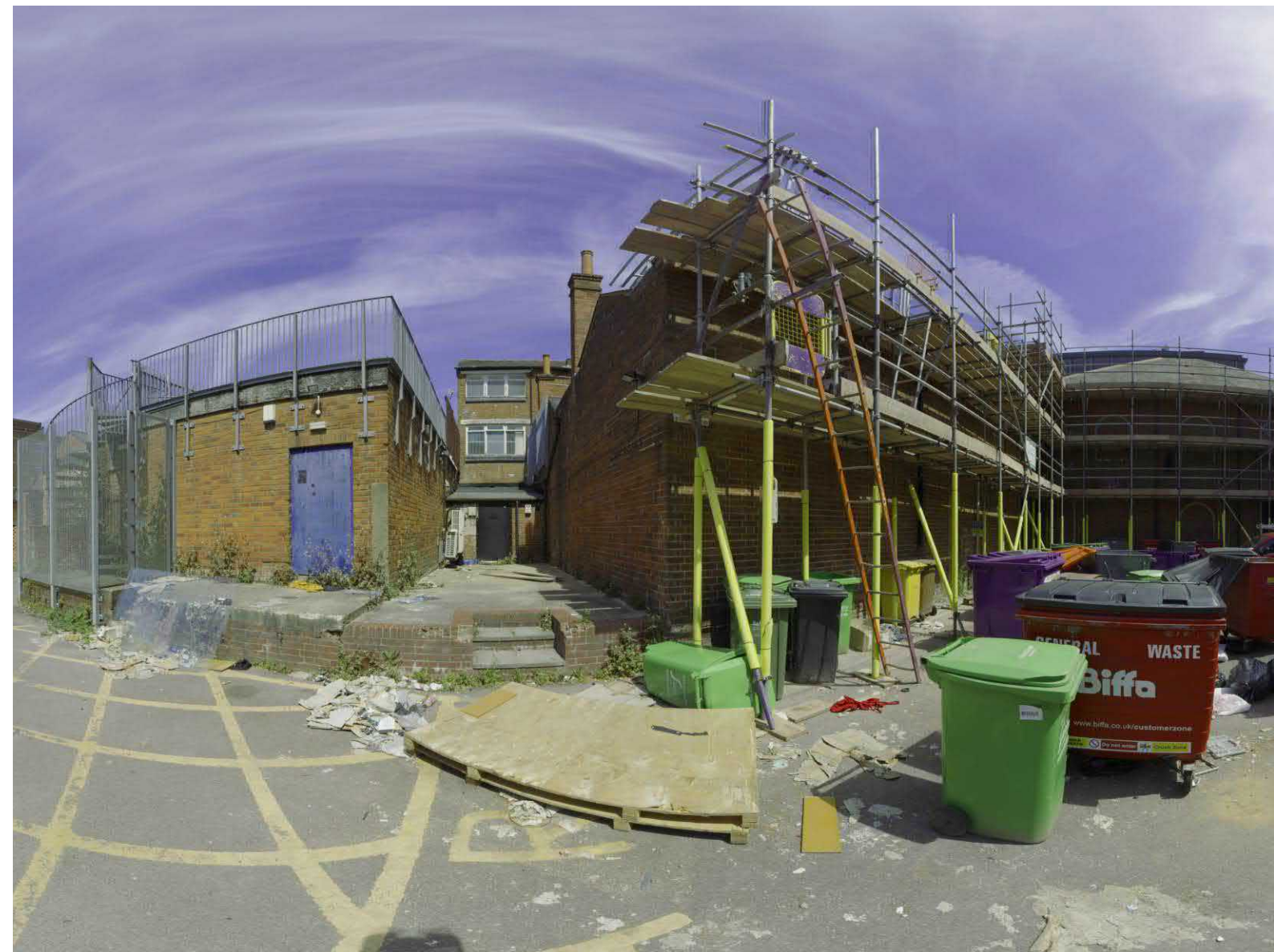
Photograph of existing unsightly rear service area
