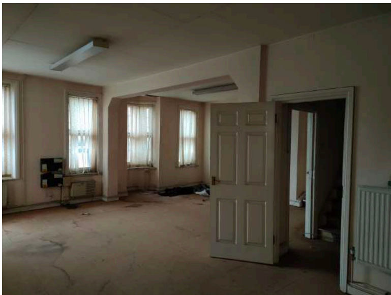
15. Second floor; main office with knock through
