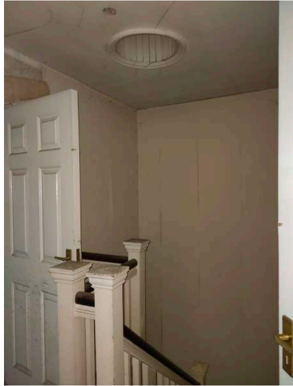
32. Third floor staircase with skylight/ventilation shaft.
