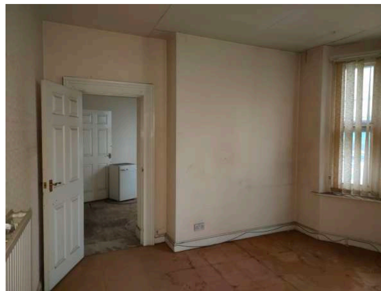
18. Second floor; link to offices
