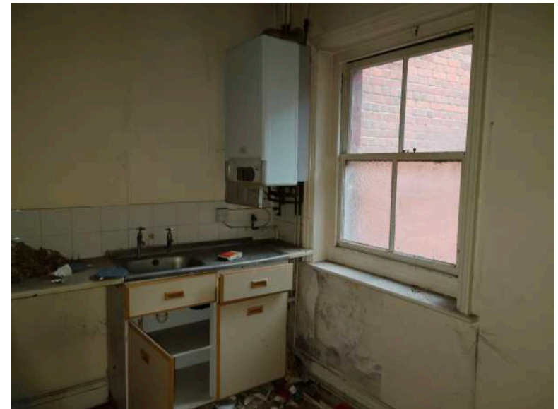
22. Second floor kitchenette in lobby area
