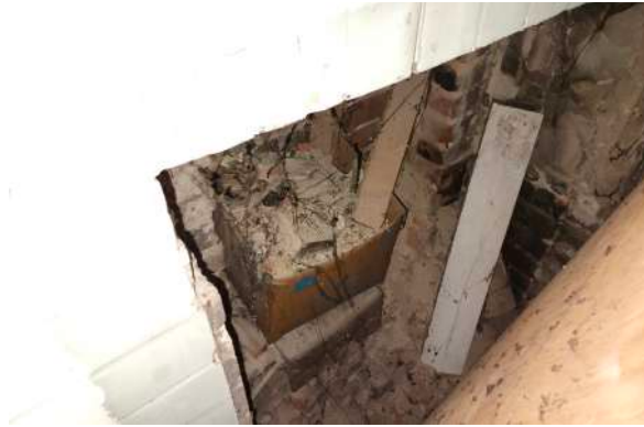
26. Blocked and remove fireplace room 1.7
