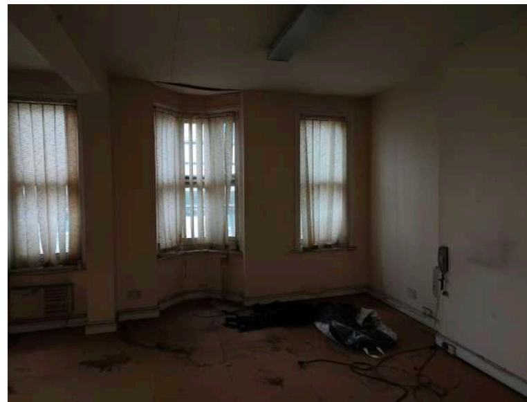
16. Second floor; former front room
