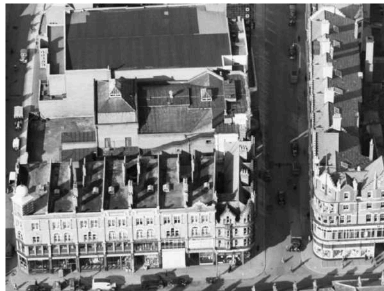
3. The application site; EAW034975 ENGLAND (1951)
