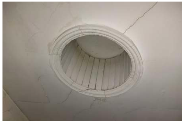
34. Third floor main staircase skylight
