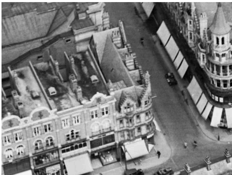
2. The application site; EPW022700 ENGLAND (1928)
