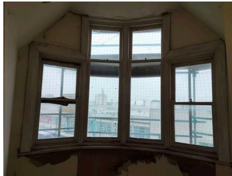
24. Third floor; window in corner gable room 3.6 on plan
