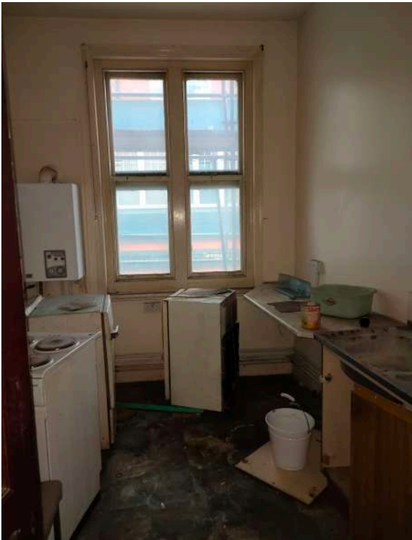
12. First floor; kitchen
