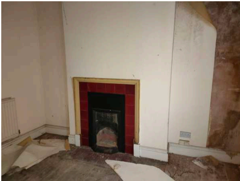
21. Second floor; fireplace in room 2.1
