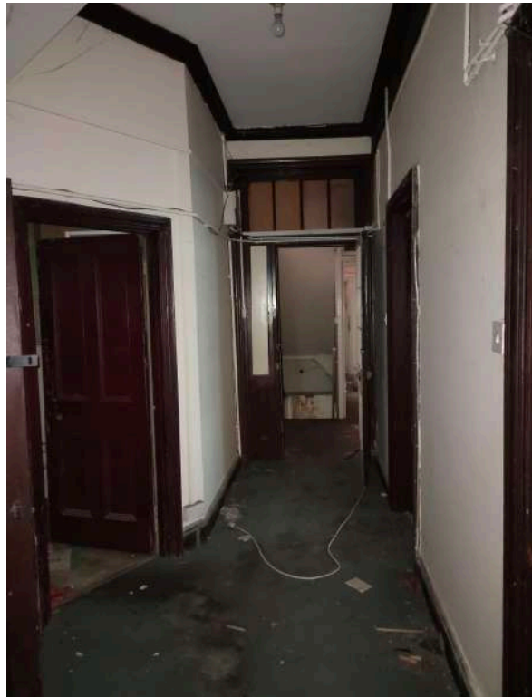
13. First floor lobby
