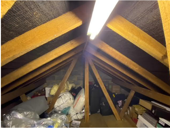
Photograph 12 – Eaves facing south-east
