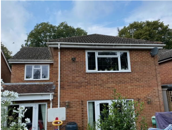
Photograph 9 – Roof facing South
