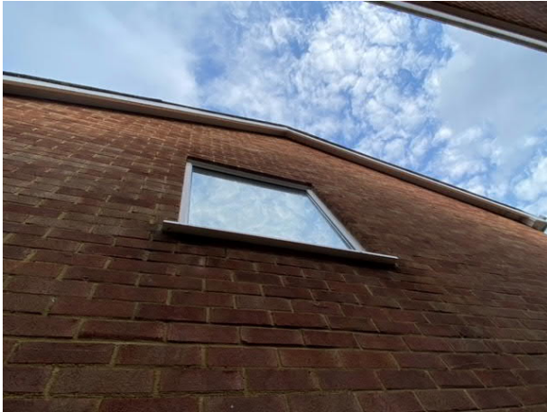
Photograph 6 – East Elevation with extension
