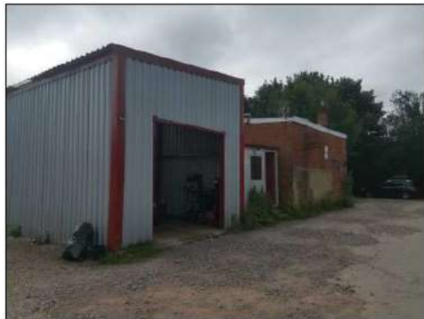
Motor repairs garage on eastern section
