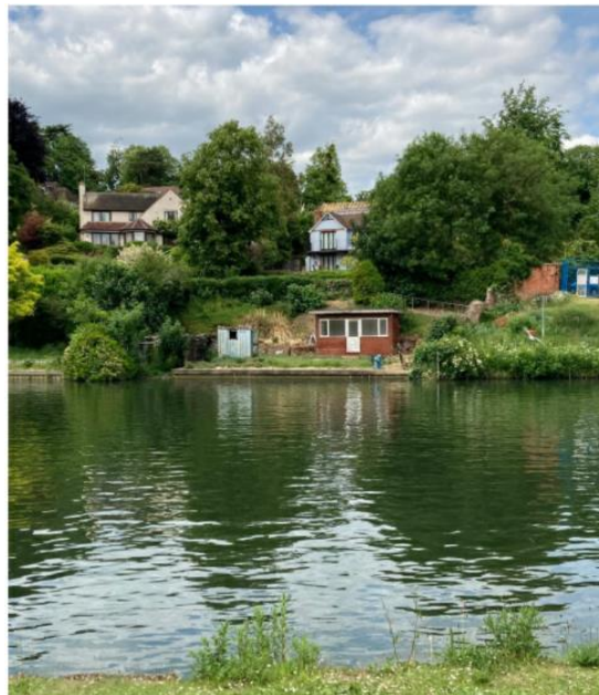
The application site with existing buildings
