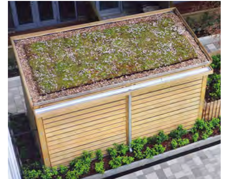
Timber cycle lockers with green roof
