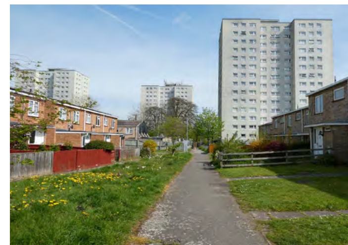
Approach View 6 : Wensley Loop (Facing West)
