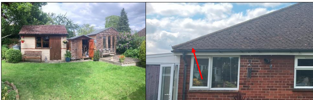
Photograph 3a (left) & 3b (right). Left – The outbuildings with negligible bat roosting potential in the rear garden of 2 Send Road. Right – The small area of six lifted tiles on the south-eastern corner of the bungalow roof which require licensed ecological supervision of the tile removal prior to any mechanical demolition.
