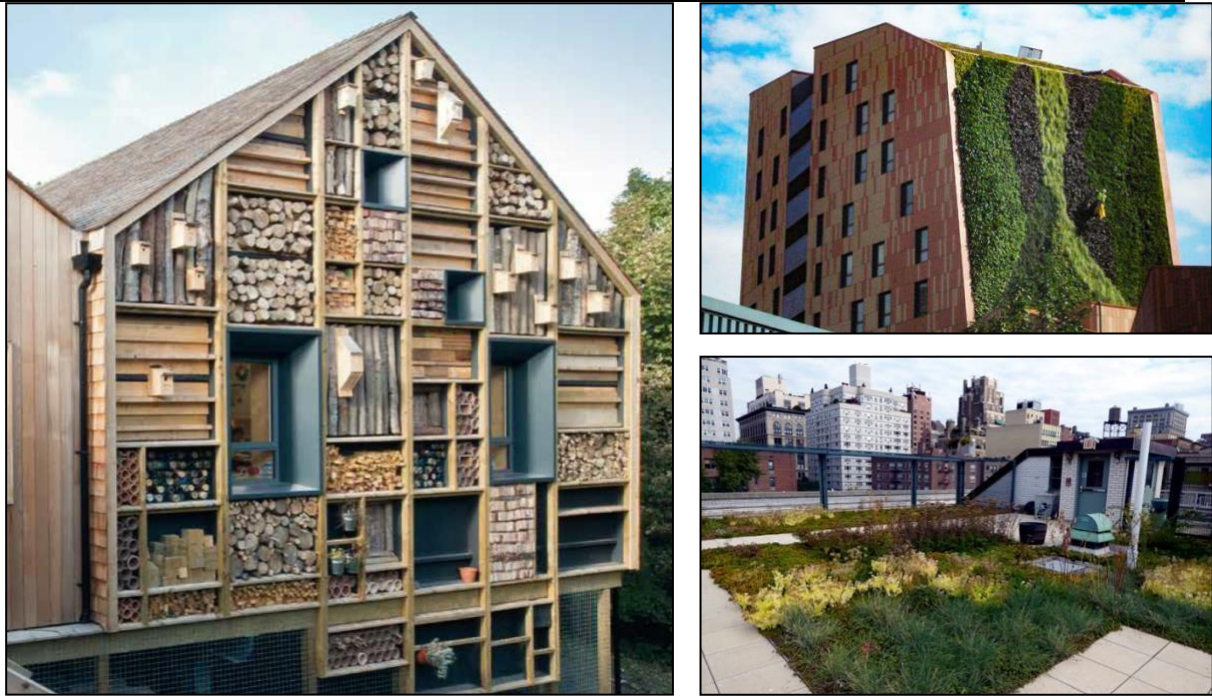
Figure 6a (left), 6b (top right) & 6c (bottom right). Left – Example of a habitat wall built to encourage birds, bats and invertebrates. Top right – Example of a living wall. Bottom Right – Example of green roof planting.
