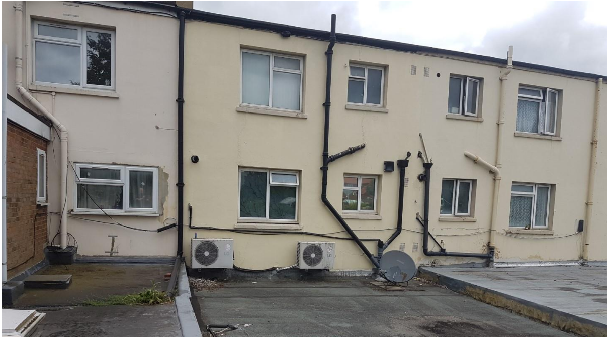
Figure D3 – Photo highlighting adjacent commercial rooftop plant, adjacent rear elevation.
