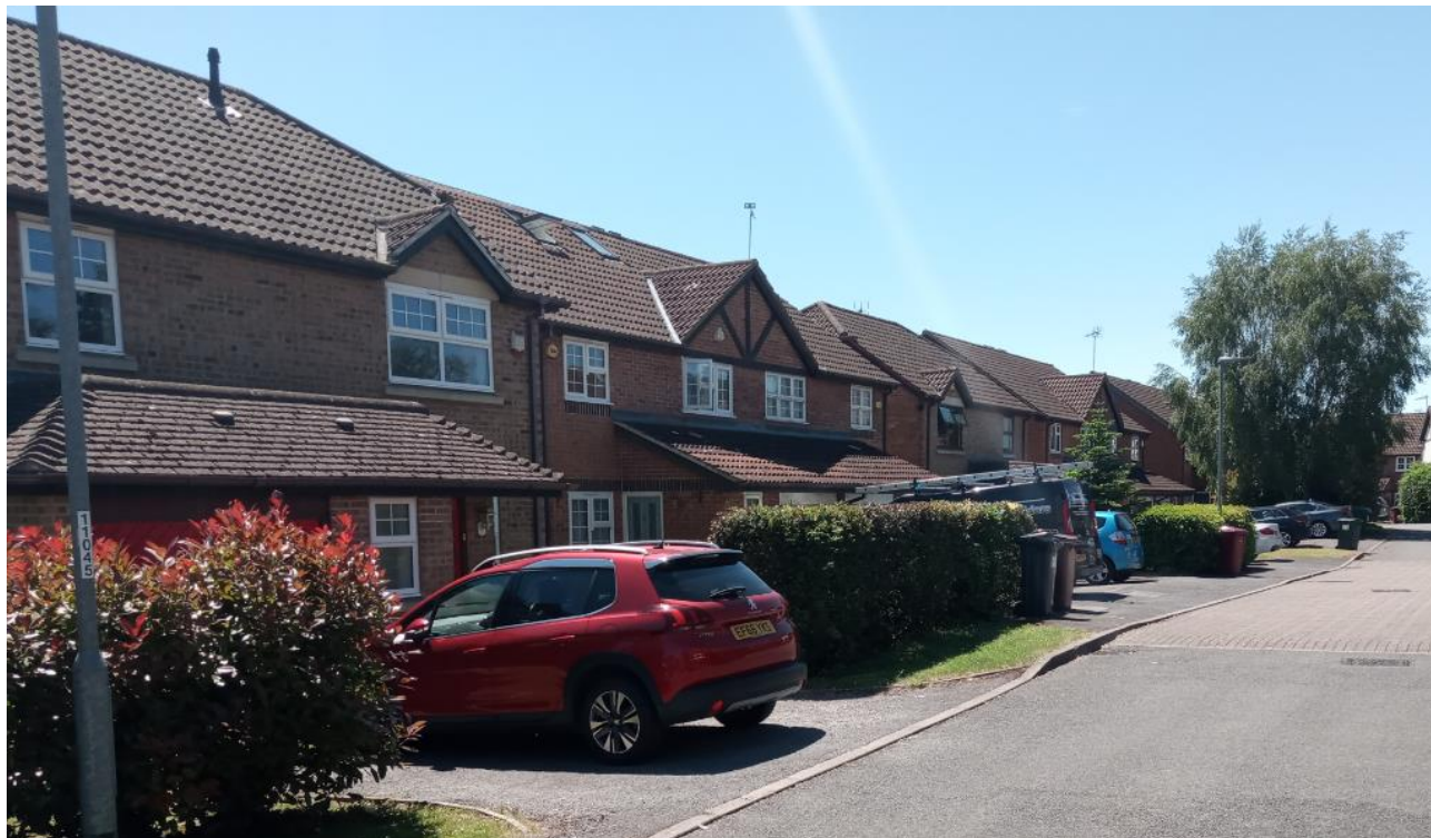
Officer site photographs of the application site property during an unaccompanied site visit on 09/06/2021.
