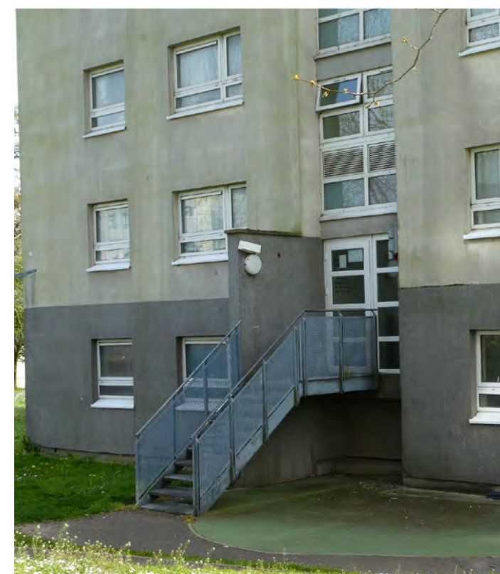
Riversley Court - First Floor Fire Escape
