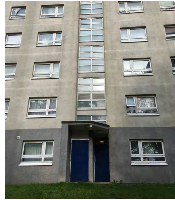
Riversley Court - Ground Floor Fire Escape
