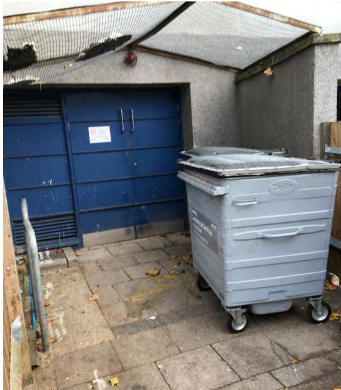
Wensley Court - General Waste Area
