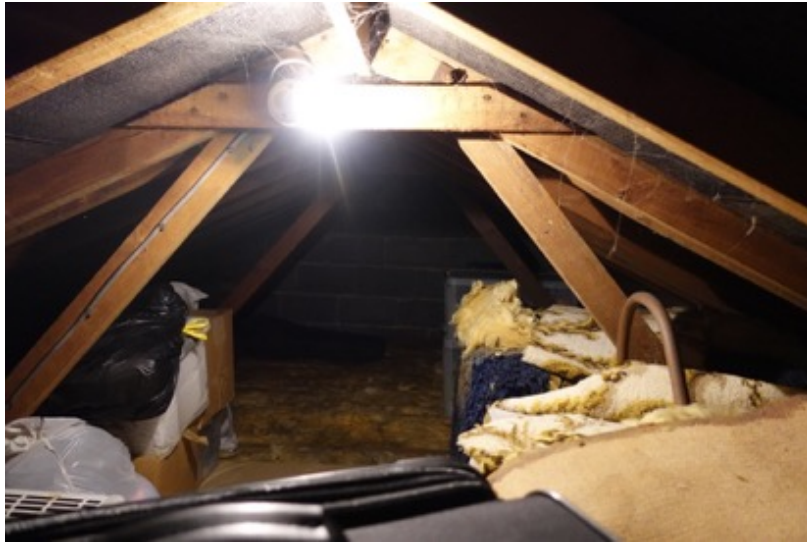
Plate 5: Inside the Loft Space
