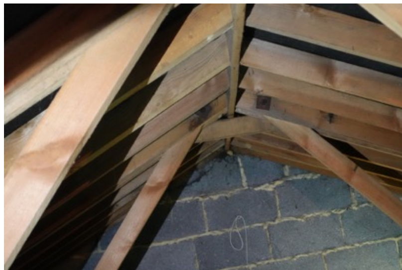
Plate 6: Timber Roof Trusses and Breeze Block Gable Ends
